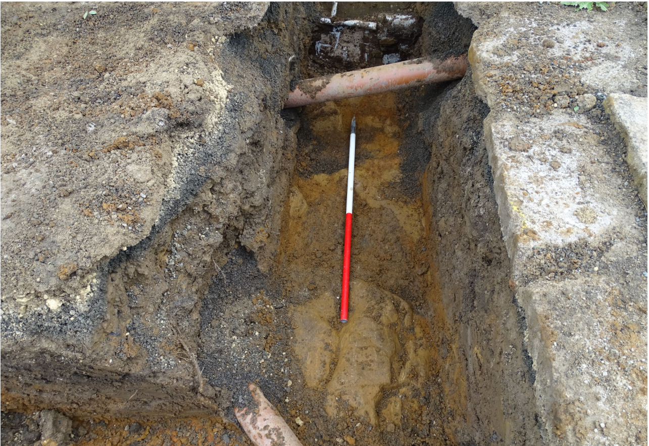
Plate 5. The southern trench leg looking east
