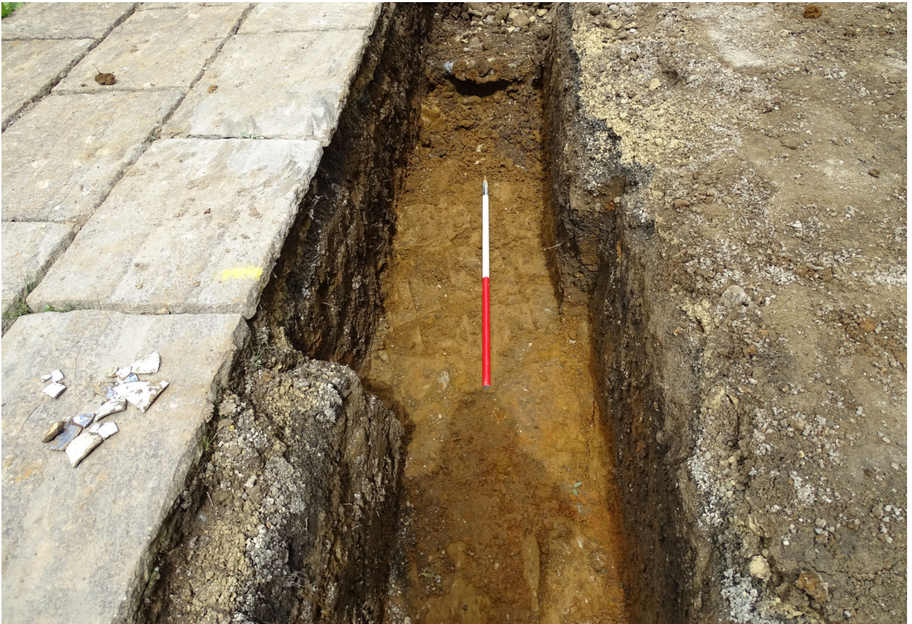
Plate 3. The western trench leg, northern half looking north during excavation
