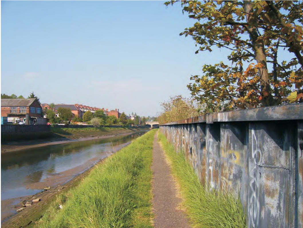
Pl. 7 Path beside the existing flood wall beside the river (looking west).
