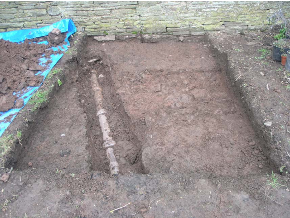
Figure 6: Looking north showing pipe trench (504)
