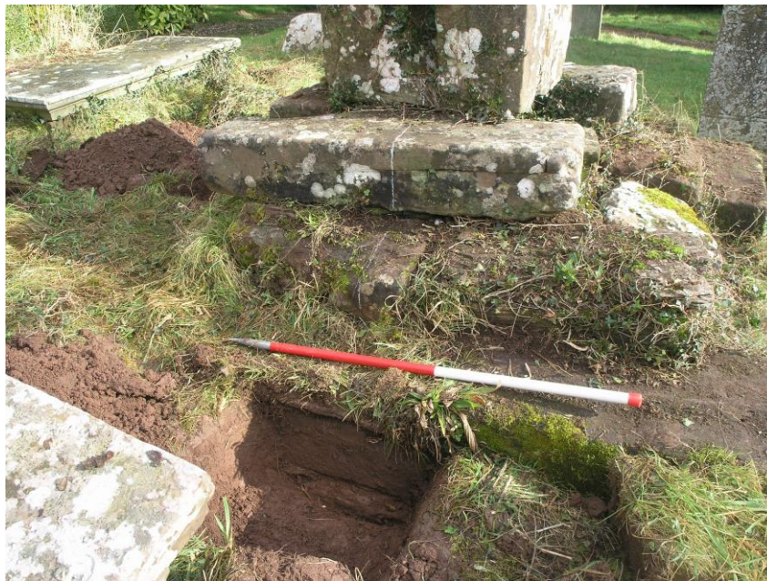
Plate 8: Western face of cross base, looking east, showing well coursed large block foundation
