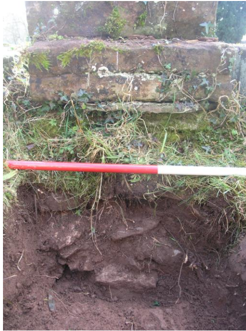
Plate 2: Northern face of cross base, looking south, showing un-coursed rubble foundation.
