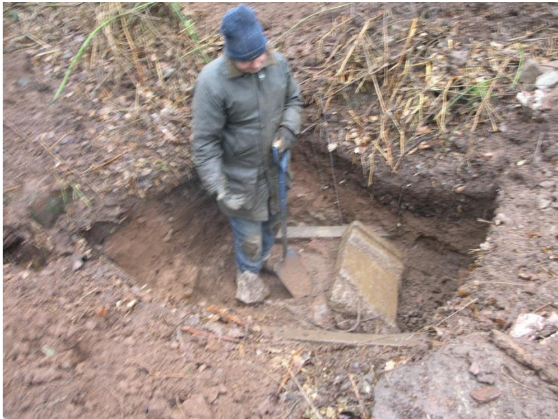
Plate 1: Reinforced concrete blocks and other remains under excavation.
