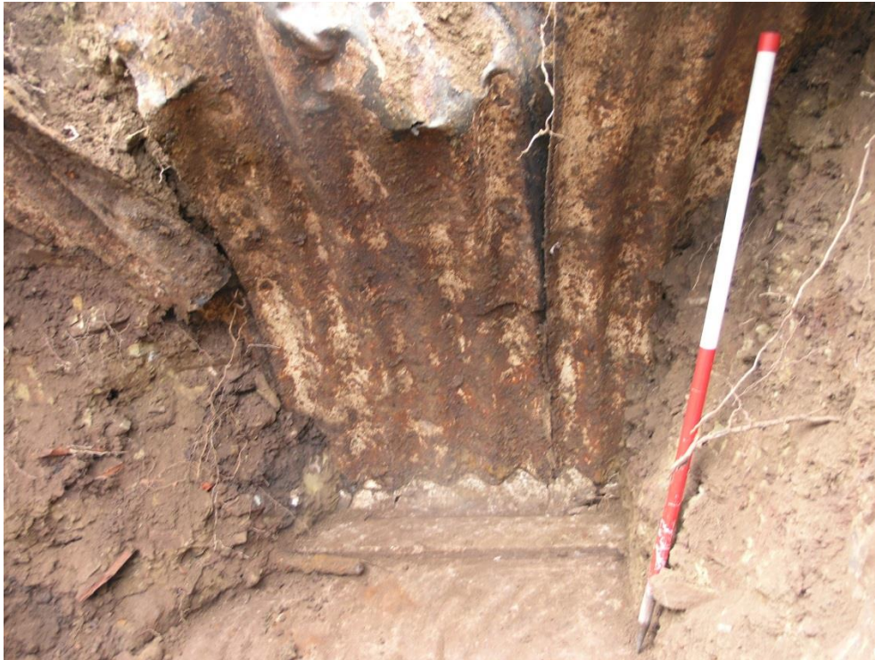
Plate 6: Detail of the wat that the concrete floor was attached to the corrugated iron superstructure, showing the cast "step" and the concrete fillet.
