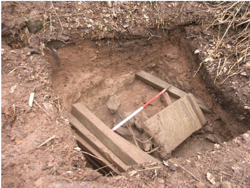
Plate 2: OB1 entrance shaft remains showing the concrete beams lining of the shaft which is cut into bedrock.
