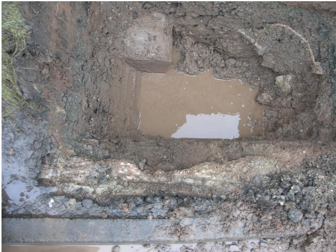
Plate 3: Trench "in plan". The squared corner represents the south-western corner of an inspection chamber.
