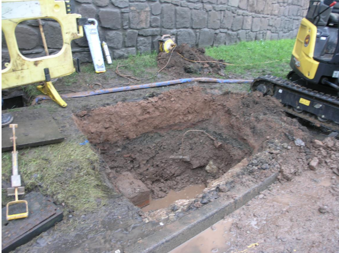
Plate 4: Trench at finished depth showing a well mixed, modern layer of disturbance containing concrete, walling stone, brick and off cuts of reinforcing wire.
