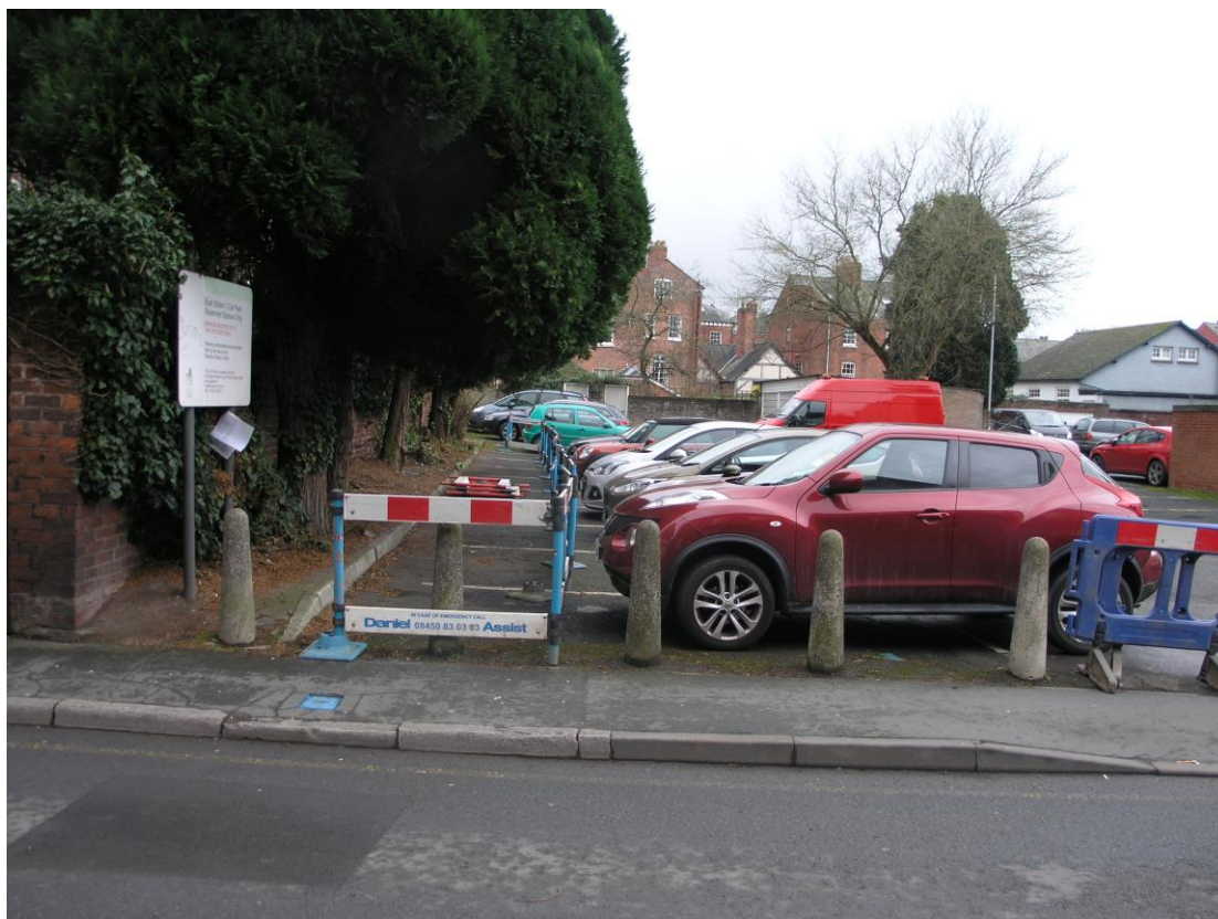
Plate 1: View southwards along line of works.
