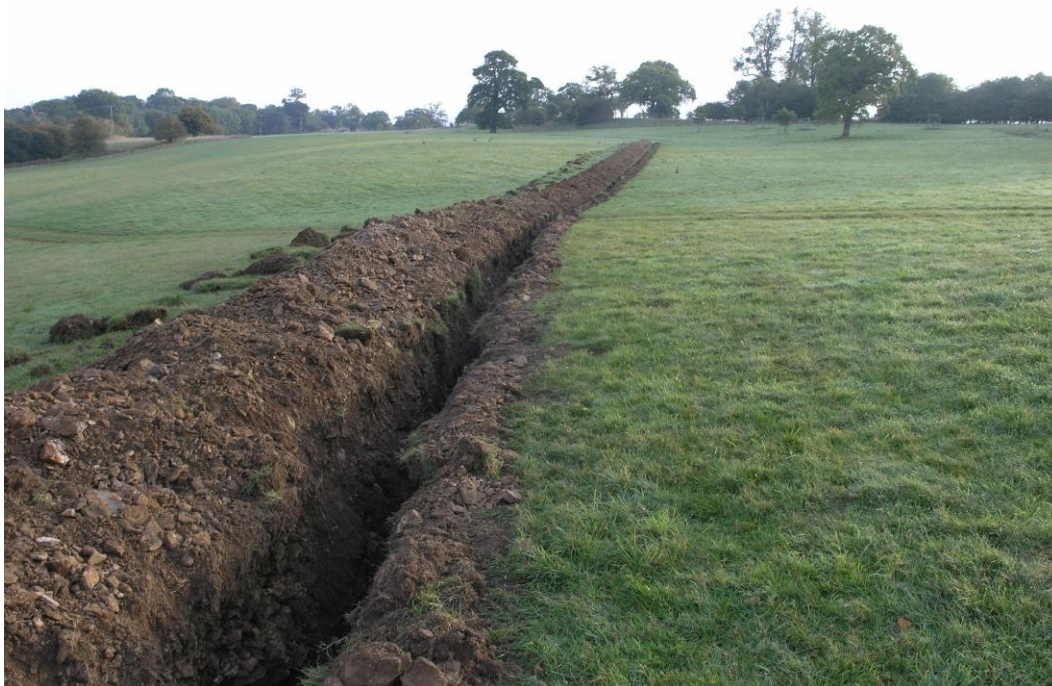
Plate 1. Cable trench looking from the track, upslope to the north-east..
