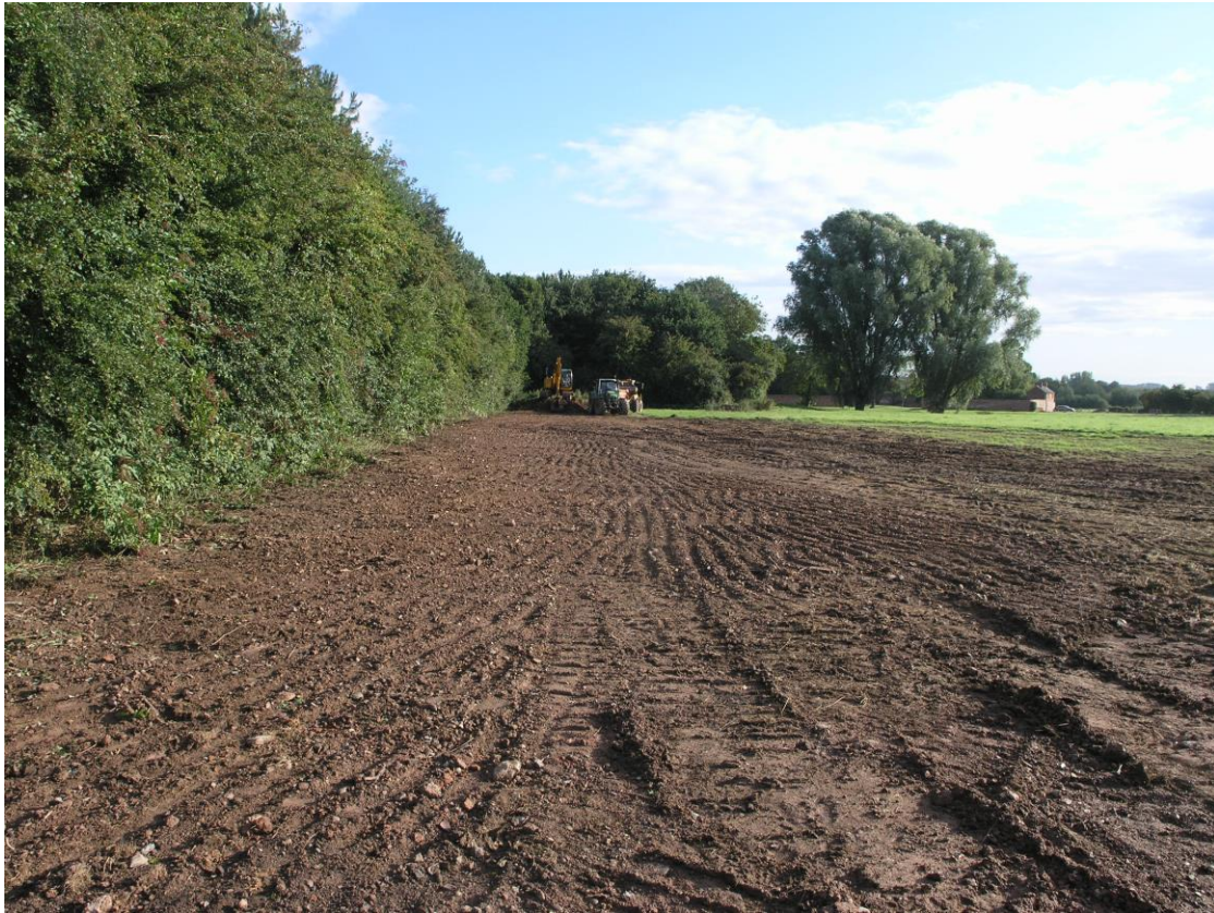
Plate 6: Removal of material along western boundary after initial harrowing / topsoil spreading.
