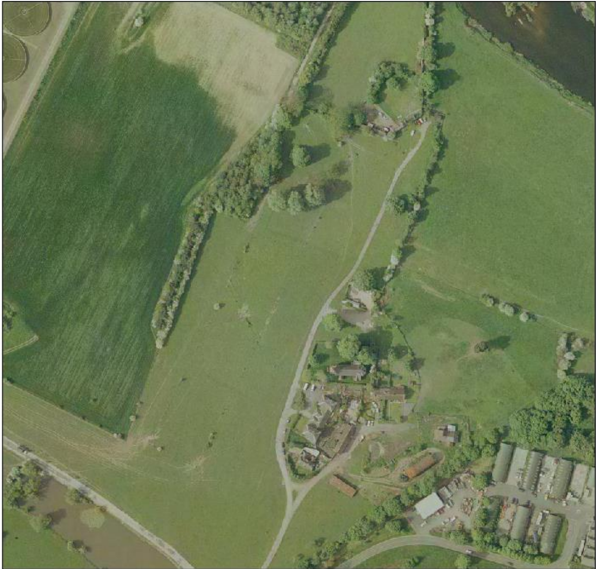
Figure 4: Aerial Photograph of 2000 showing retained parkland and lack of southern boundary to site. © Crown copyright. All rights reserved 100024168.
