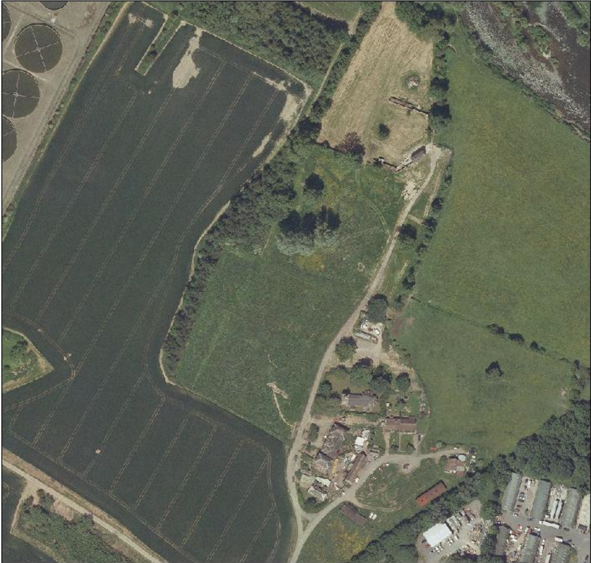
Figure 5: Aerial Photograph of 2009 showing new, straight southern boundary, parkland under cultivation and scar for a replacement water main. © Crown copyright. All rights reserved 100024168.
