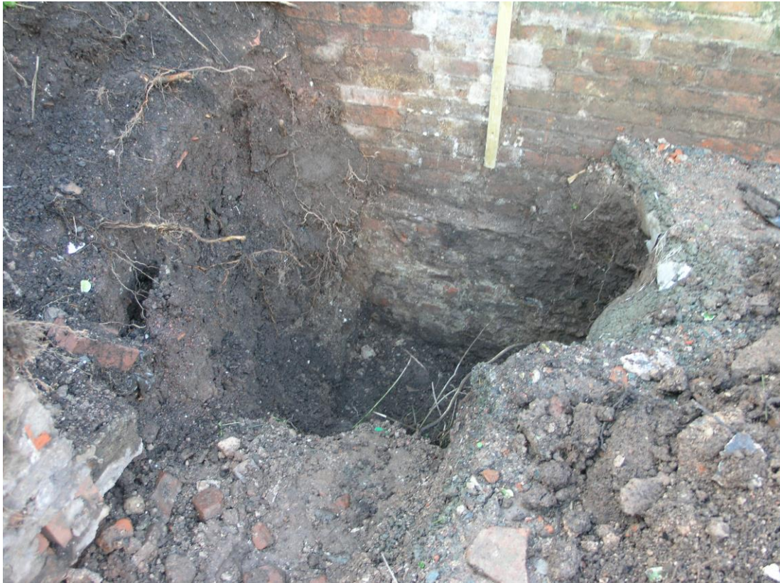
Plate 3: Trench looking south.
