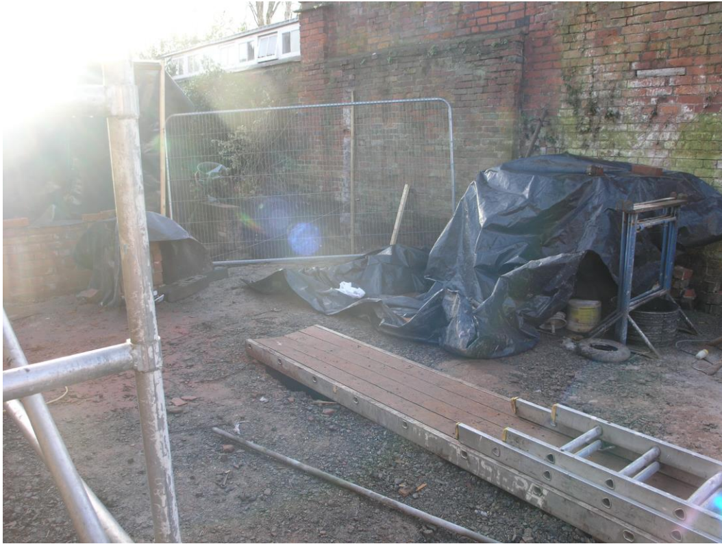
Plate 1: Trench looking south-east
