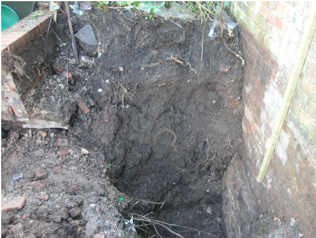
Plate 2: Trench looking east.
