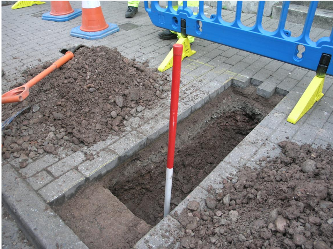
Plate 1: Trench 1 looking north-east
