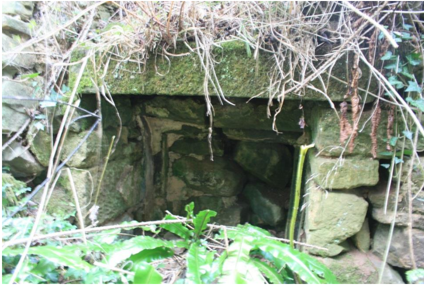
The east wall (exterior); cupboard-like feature at south end
