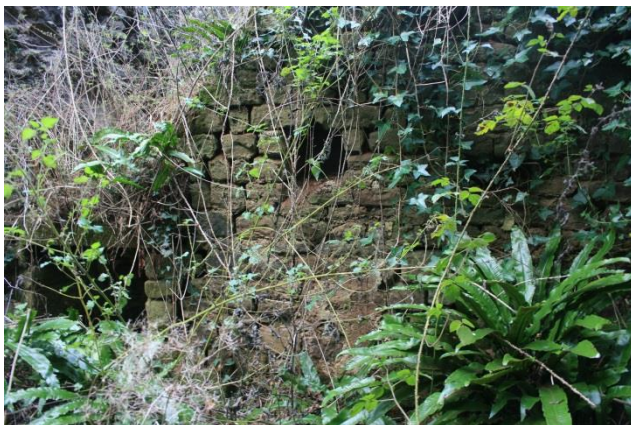
The east wall (exterior): the south end showing different (smaller) masonry type and cupboard-type feature bottom left
