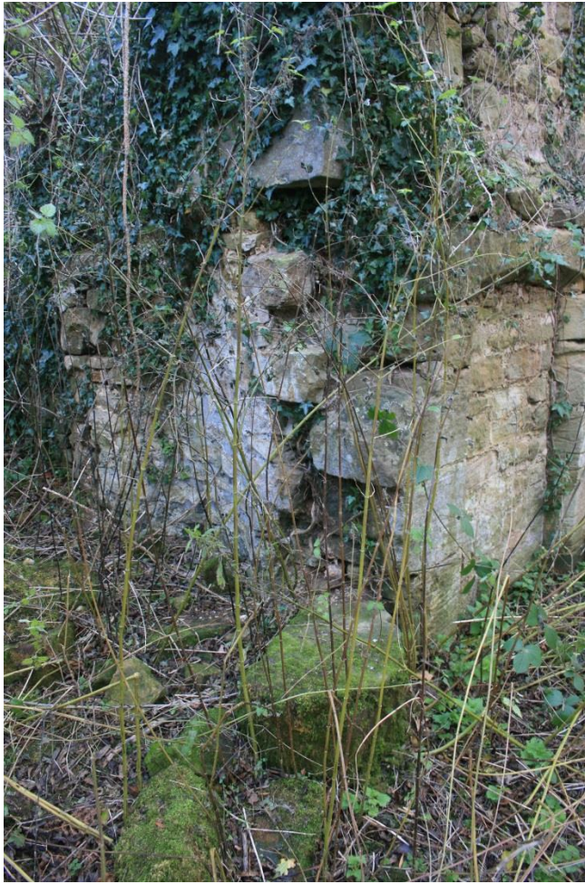
The south-west corner (exterior) showing west wall fabric with curved hollow (partly rendered). The large stone in the foreground at the corner may be an alleged column base
