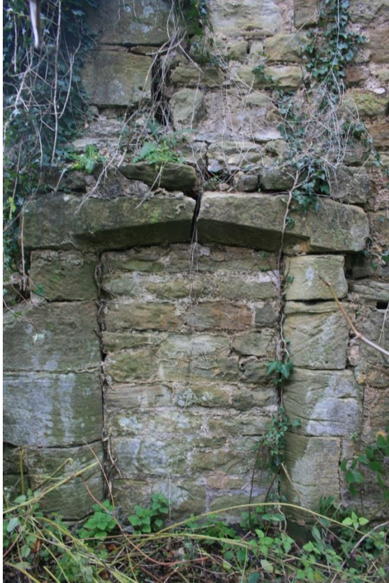
South gable wall (exterior): blocked doorway at south-west corner
