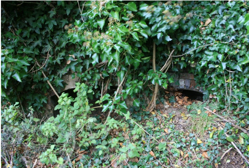
The north wall (interior): two oven openings within the NE corner
