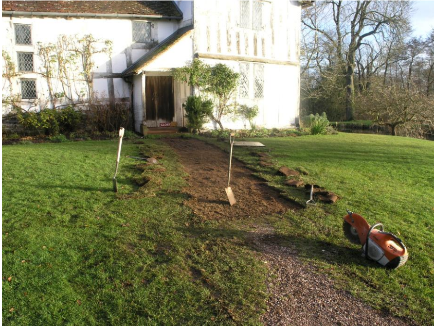
Plate 2: The path under excavation
