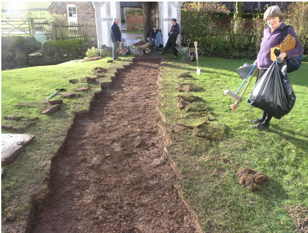
Plate 3: The excavation completed prior to the laying of mortar and flagstones.
