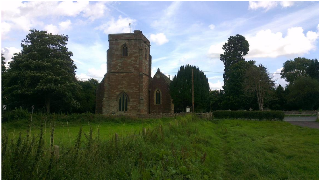
Figure 15: St Bridget's Church viewed from the west. The small enclosure identified as containing the Tithe Barn is in the foreground in the right of the picture. © Herefordshire Council
