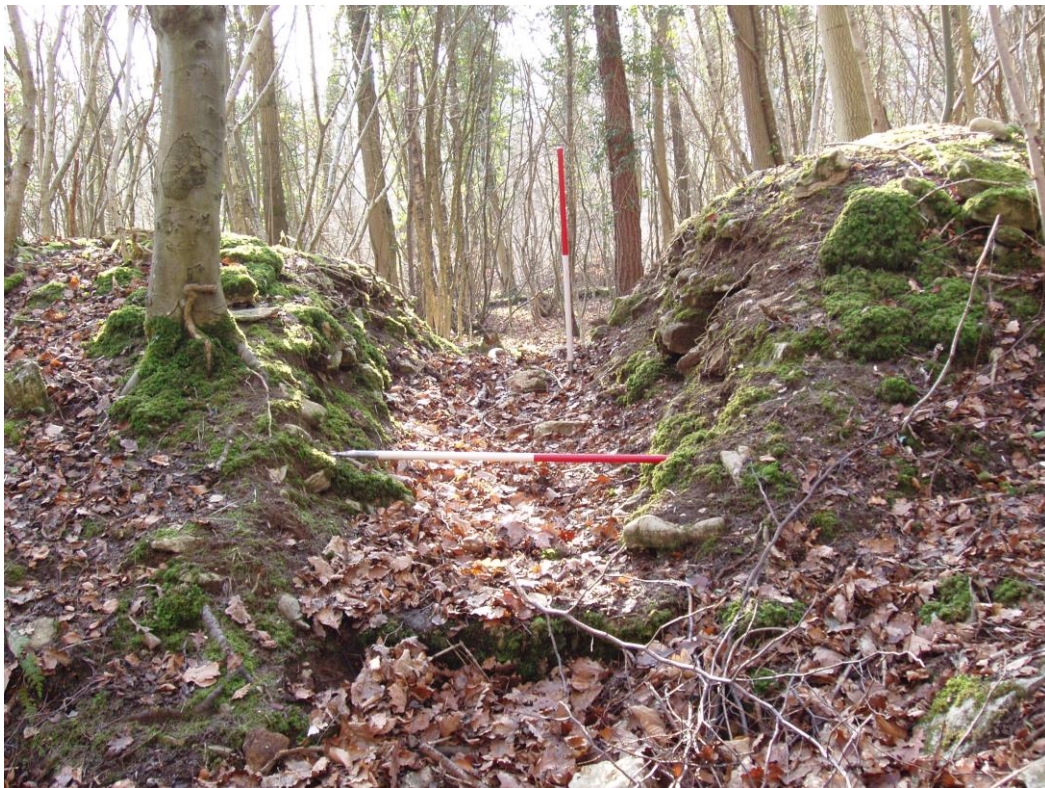
Plate 4: Trench C showing the continued erosion of the inner rampart from the northeast.
