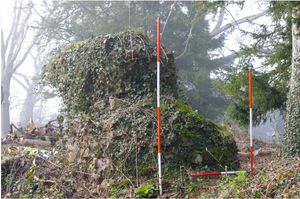
Plate 22: View of the Stair Tower from the northeast before work began.
