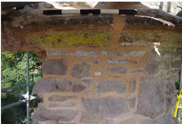
Plate 11: Area beneath the moulding after consolidation.
