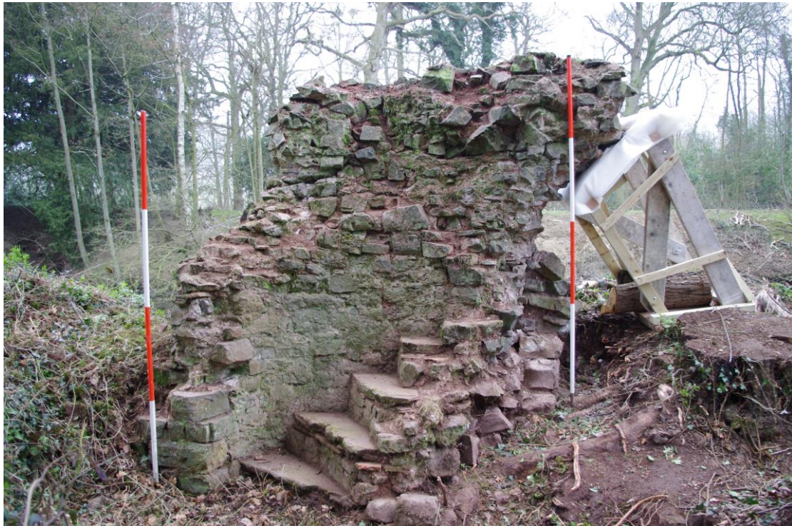
Plate 19: View of the Western elevation of the Stair Tower from the southwest after it had been cleaned and the over-hang supported.
