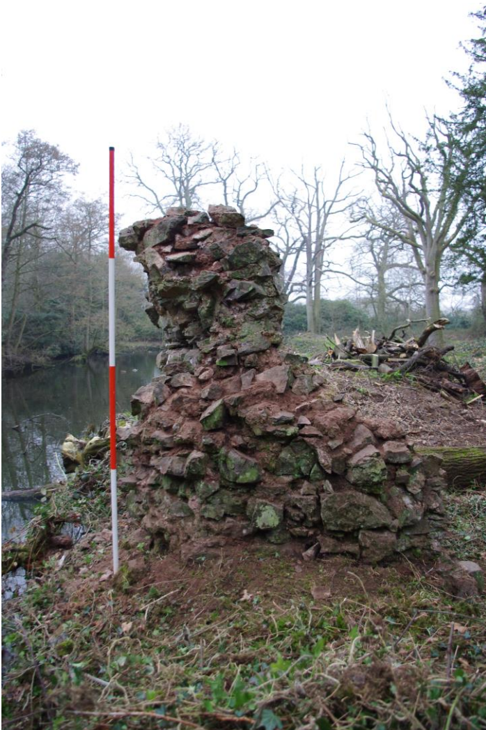
Plate 25: View of the Stair Tower from the north after vegetation removal.
