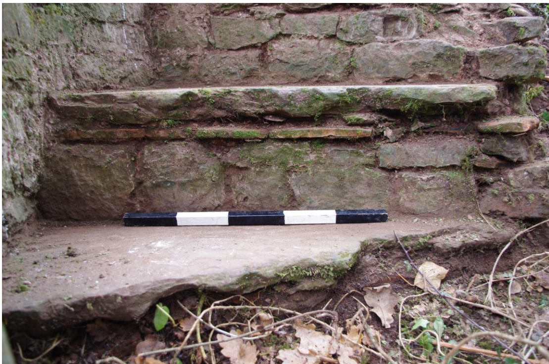
Plate 21: Third step from the top showing the insertion of a tile layer.
