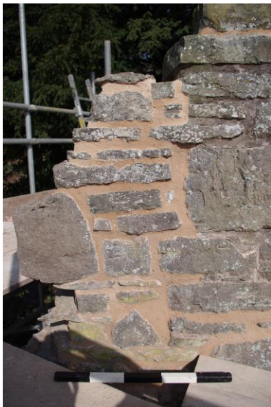
Plate 9: Upper portion of the gatehouse tower after completion as seen from the southwest.
