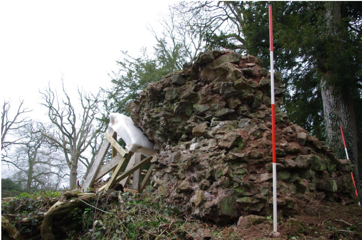
Plate 23: View of the Stair Tower from the northeast after the vegetation had been removed.
