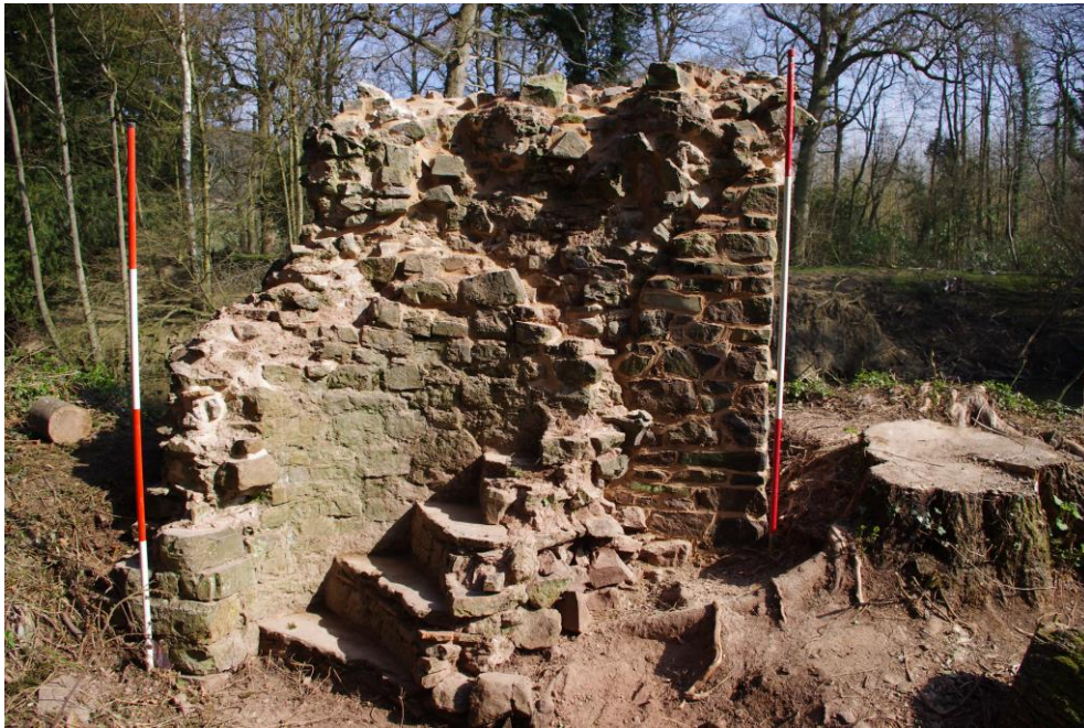
Plate 29: The completed stair tower after pointing and the addition of the support wall.
