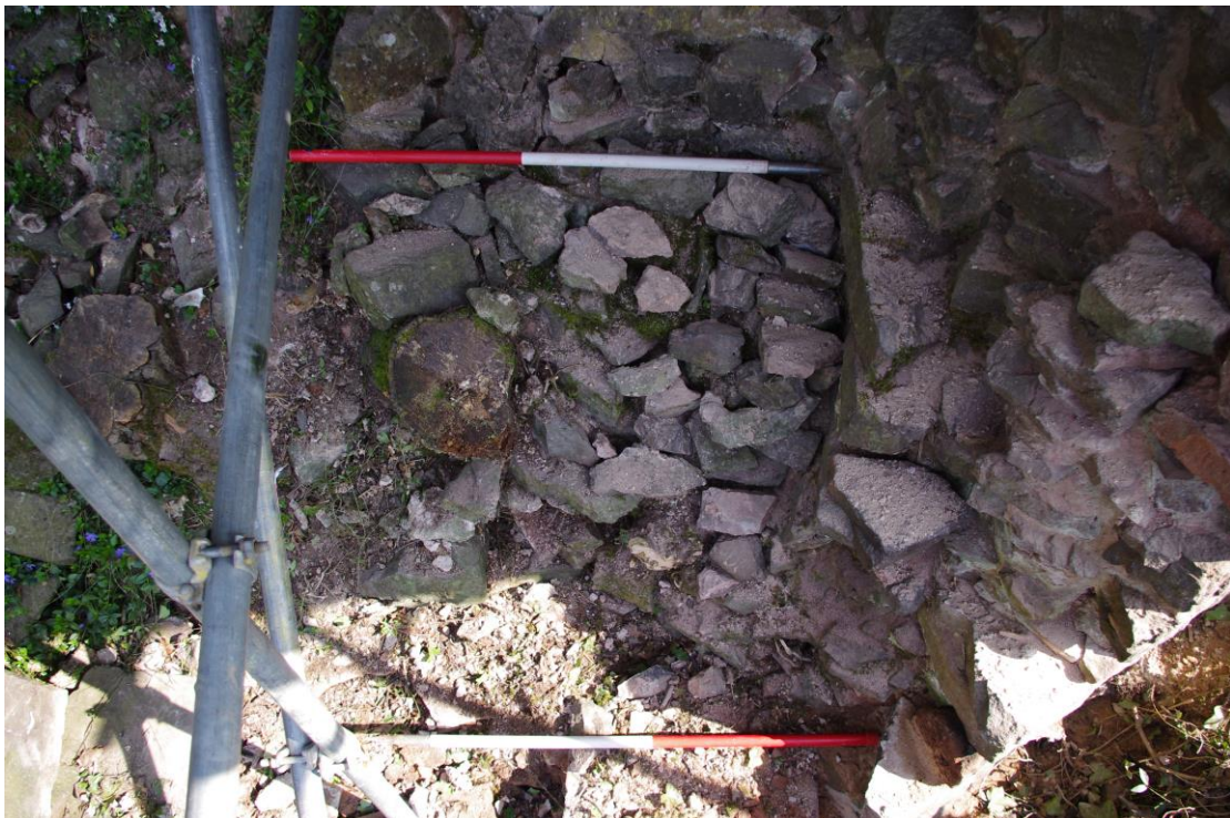
Plate 15: Gatehouse core work from above, before consolidation.
