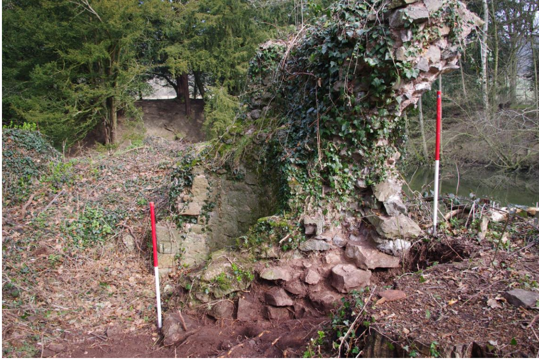
Plate 27: South facing elevation after the trench was excavated.
