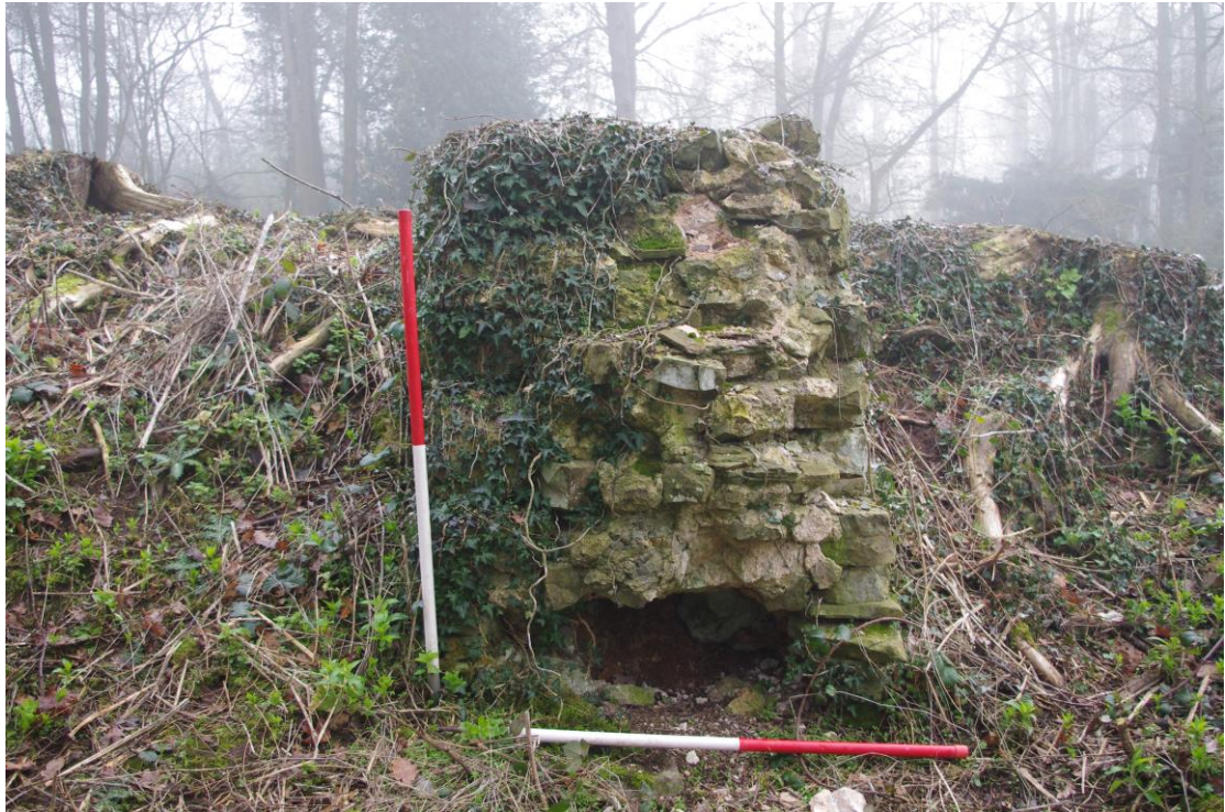
Plate 35: West facing section before cleaning.
