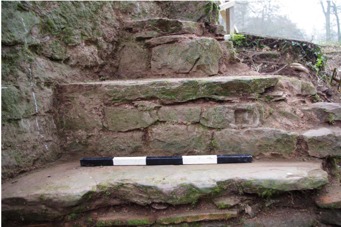
Plate 20: First and second (from the top) steps showing stone construction.
