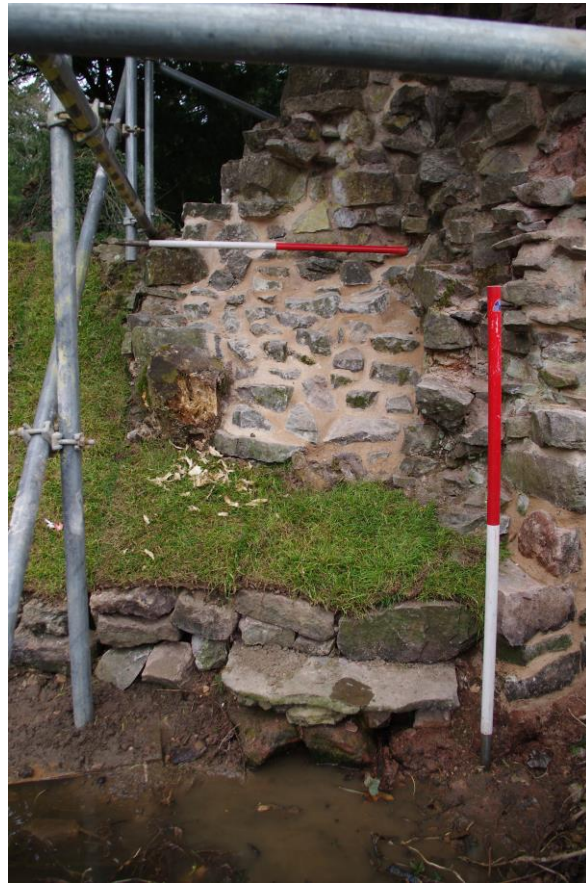
Plate 16: Corework upon completion of the project as seen from the west.
