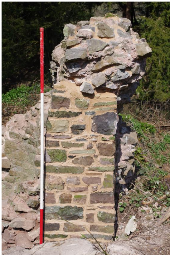
Plate 30: View of the completed support wall as seen from the south.
