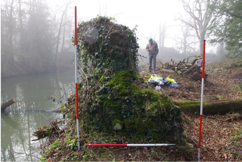
Plate 24: View of the Stair Tower from the north before cleaning.
