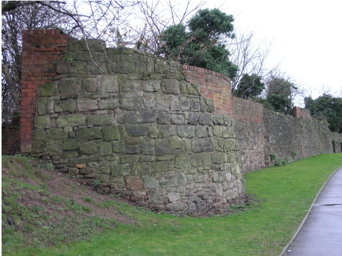
General view of section 3 looking south from Bastion 4
