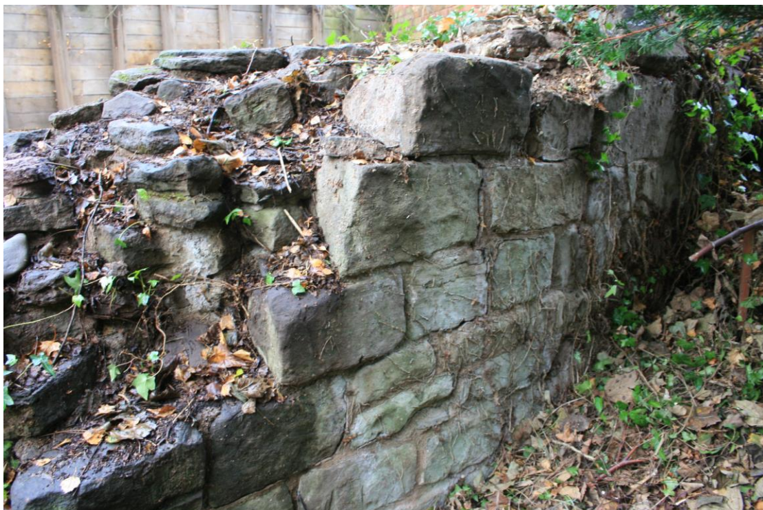
The city wall to the north of the entrance to the Cantilupe Street excavation. Excavation showed the face in this area to have been substantially rebuilt, possibly in the Civil War
