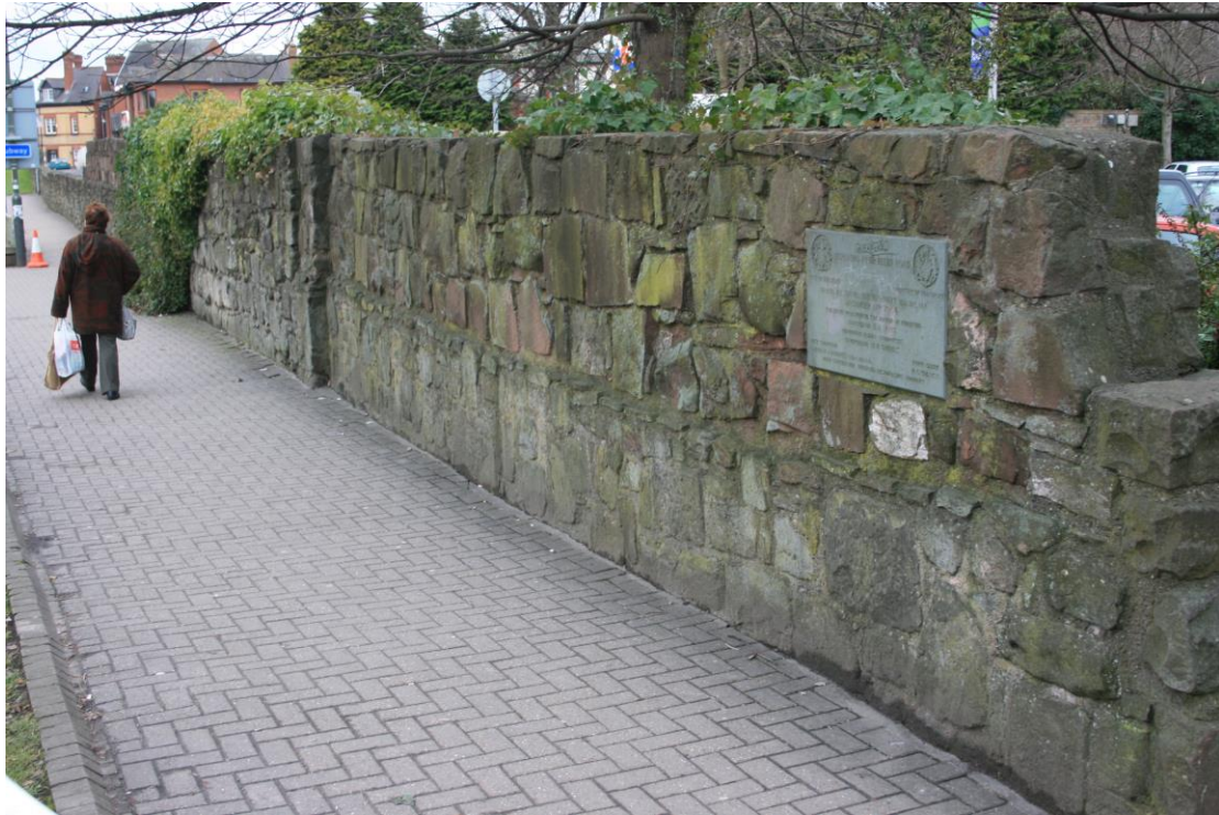
General view of the Wall Street section, looking east. The plaque in the foreground commemorates the opening of the Inner Relief Road in 1969 but is embedded in masonry of the c.1983 build. The lowest courses may be remains of the 1968 wall
