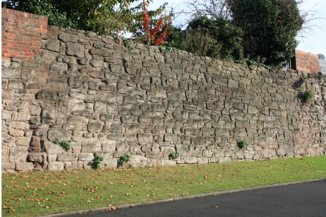
Outer face masonry of section 3 opposite the Blue Rooms plot
