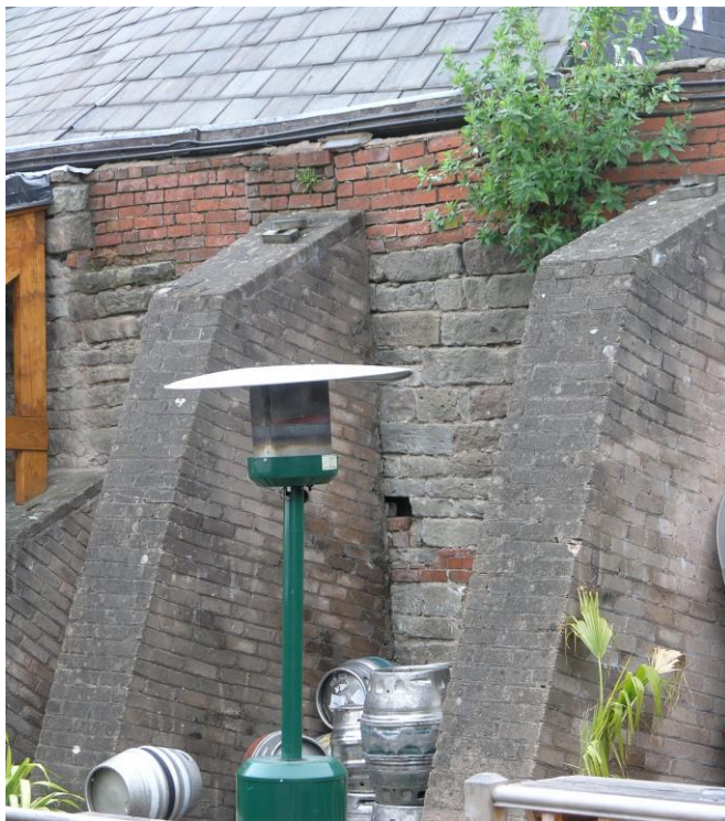
The city wall (outer face) in the yard at the rear of the Barrels pub on St Owen Street (2008). The modern buttressing hides much of the unique masonry of this section
