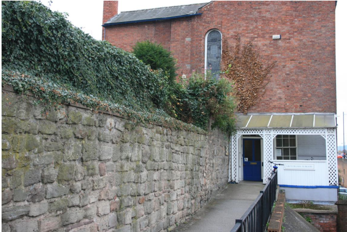
Section 2: the wall on the approach to the Greyfriars Surgery
