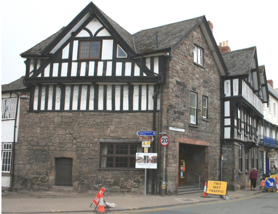
The Farmers' Club, Widemarsh Street. The lower part of the north elevation (foreground, below window-sill level) contains stonework of characteristic city wall type. The stone gable (right) would have been built to replace the end wall of the medieval Widemarsh Gate on its demolition in 1799
