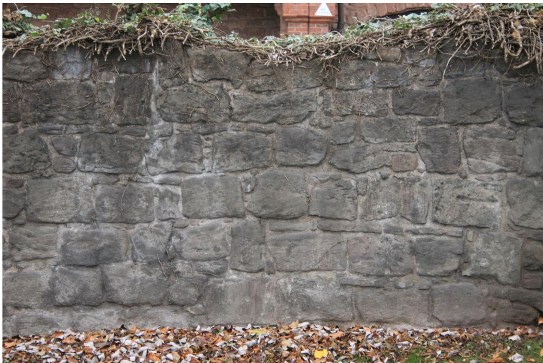
Detail of the probably primary medieval outer-face masonry
