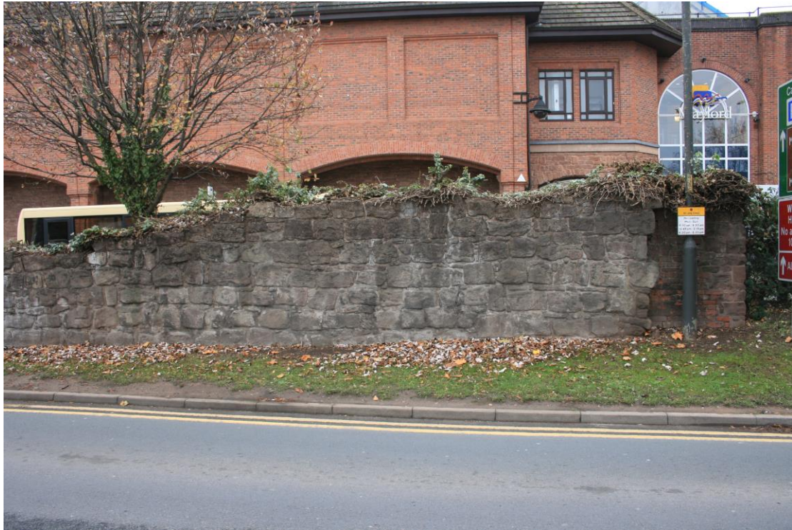
The western end of the Maylord Orchards wall, exterior face
