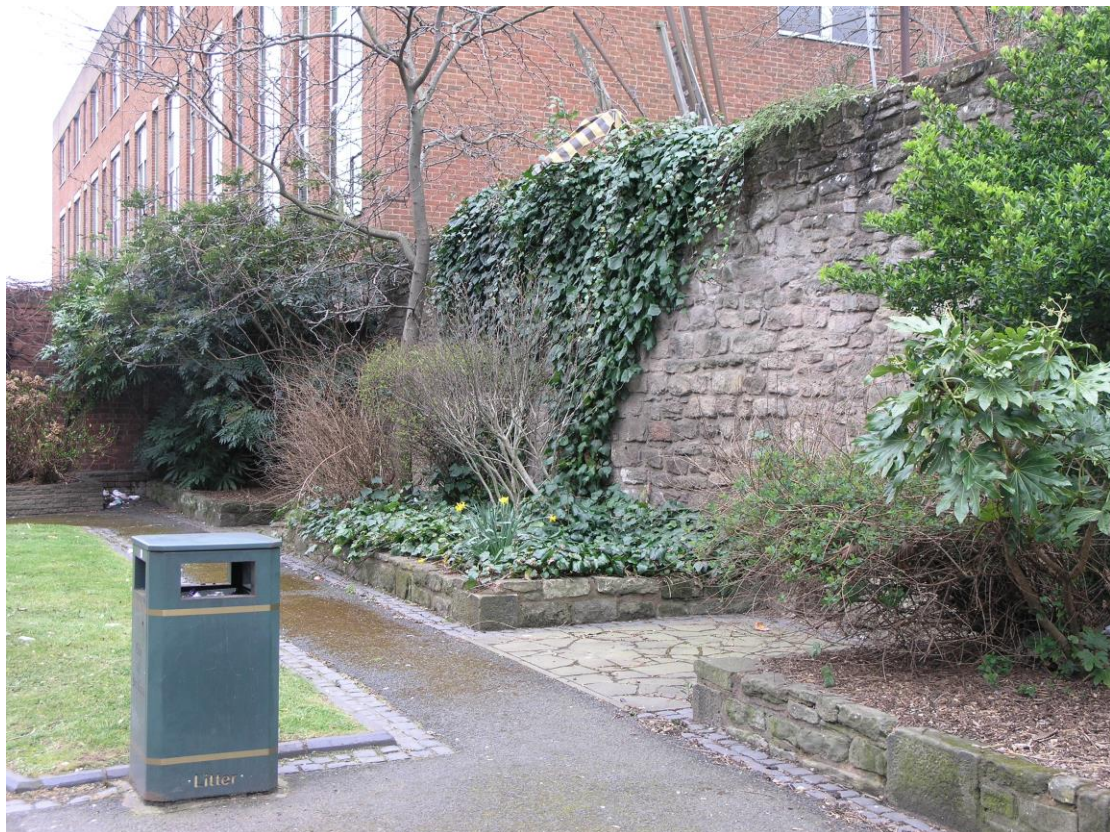
The Bastion Mews wall, east end, looking east towards the Police Station. The present (2011) electricity sub-station (overgrown wall, left) interrupts the view of the wall and disguises its continuity from Bastion Mews eastwards
