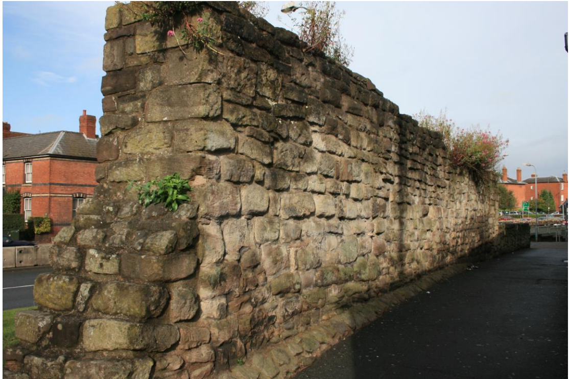
The interior face of the Gunners lane wall, looking north
