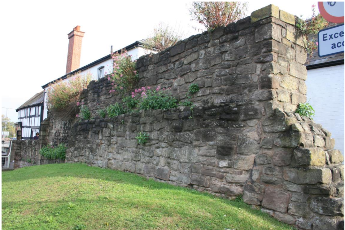
The exterior face of the Gunners Lane wall, looking north
