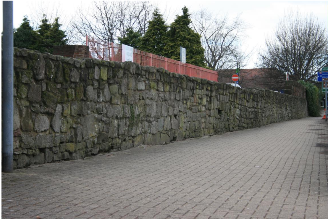
The Wall Street wall looking west alongside the New Market Street pedestrian underpass. The date of this masonry is unknown but is likely to represent a long history of ad hoc repairs in the post-medieval period with an uncertain degree of rebuilding c.1968; the blocks in the foreground may represent re-set primary facing masonry
