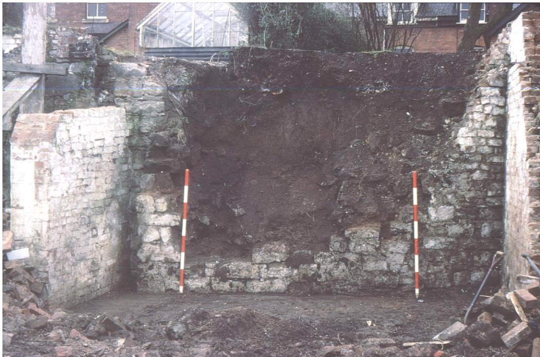
Photograph of the Mill Street – Cantilupe Street wall after removal of collapsed debris, immediately prior to excavation in 1972. (Photograph: Ron Shoemith)
