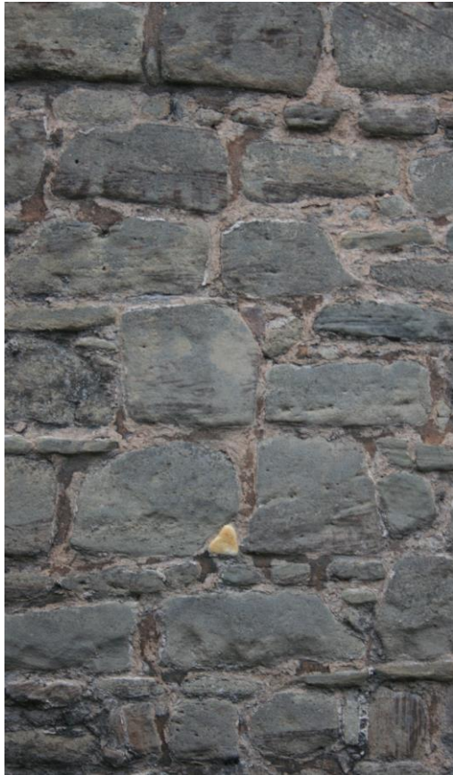
Detail of the suggested 'primary' build character masonry, seen in section 1 and elsewhere, consisting of large square blocks with short, intermittent levelling-up courses
