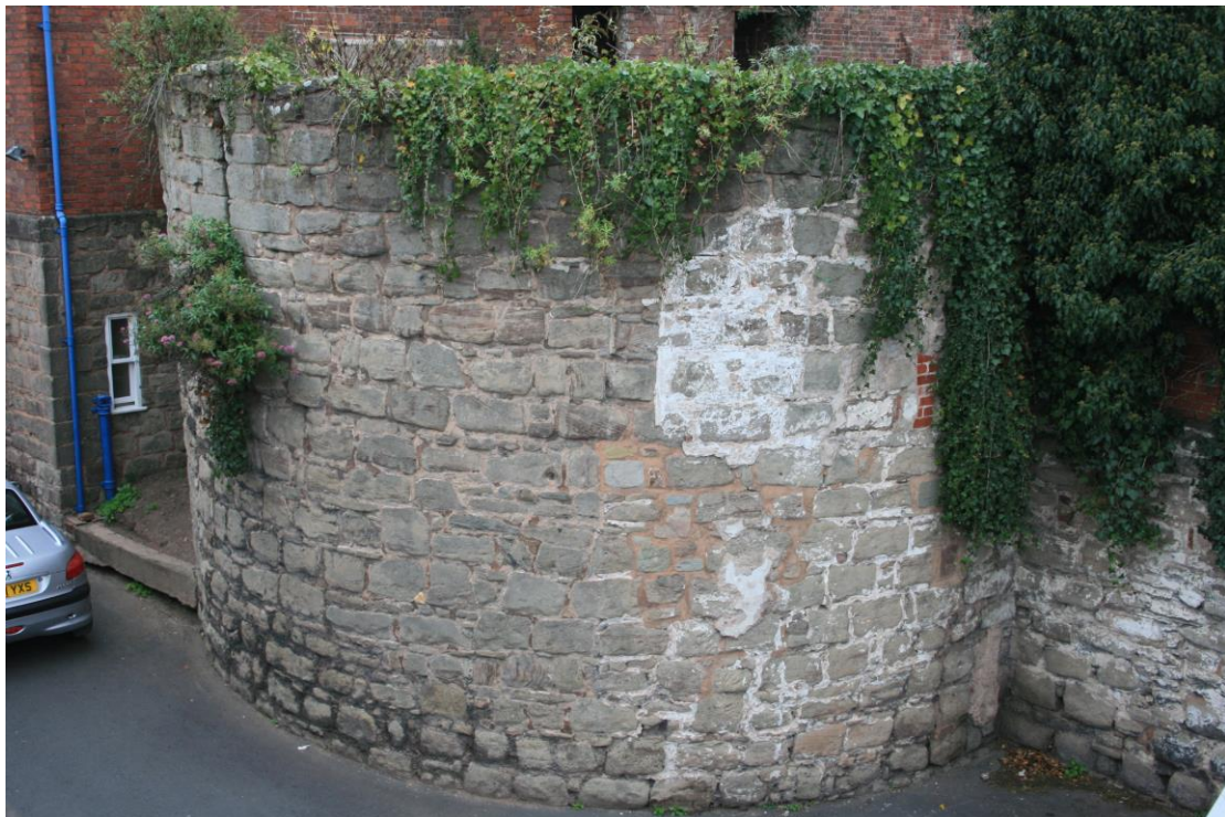
Bastion 2, adjoining the south side of the Greyfriars Surgery.
