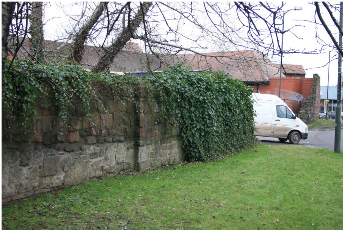
Looking west towards the north-east end of the section 7 (c.1983) wall beyond the Tesco vehicle exit. The section 8 wall in the foreground consists of base courses surviving from the 1968 wall raised by the addition of the distinctive red c.1983 Tesco-Shoesmith masonry
