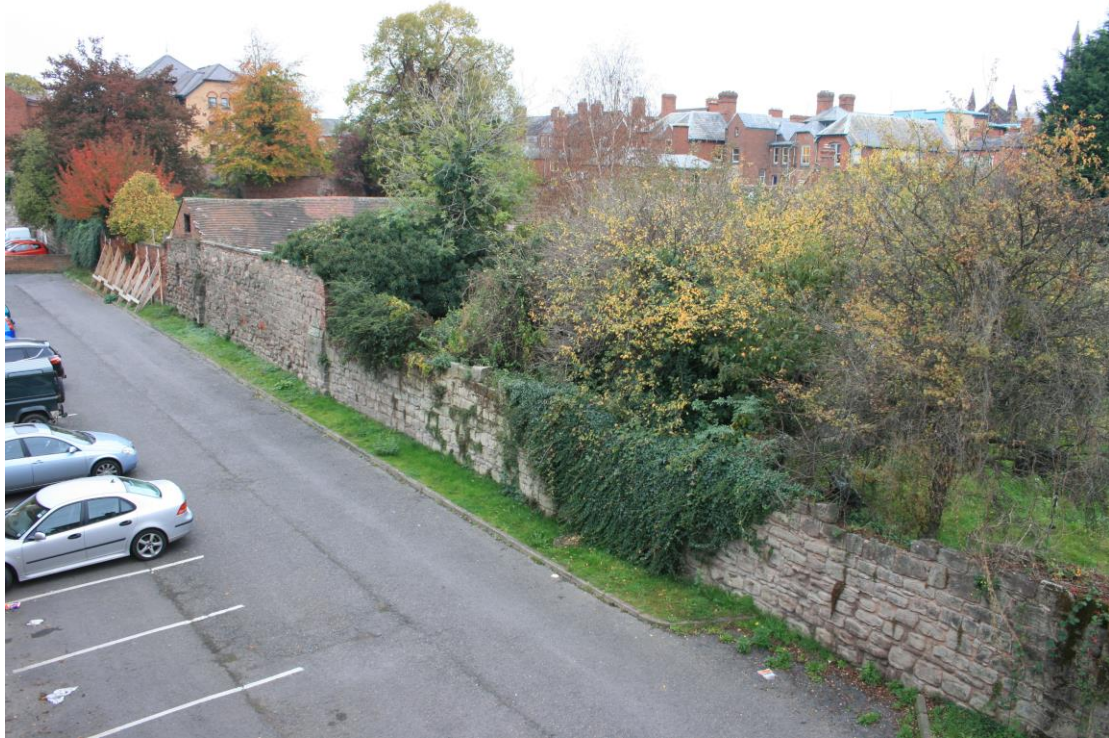
General view of the south end of section 1
