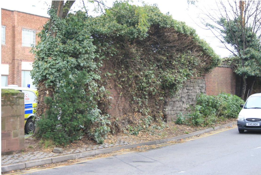
The inner face of the Maylord Orchards wall, looking east from the west end (2009). The problem of ivy, tree growth and the proximity of traffic to the wall face is apparent
