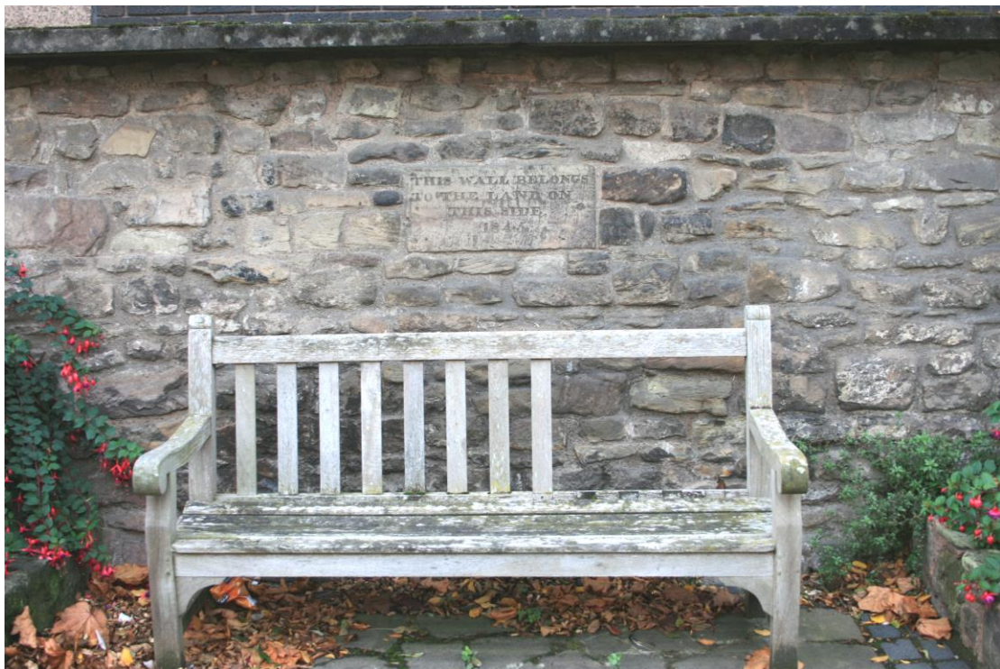
The (rebuilt) wall in front of the Bath Street Police Station. The plaque reads 'This wall belongs to the land on this side [ie the former ditch] 1845'
