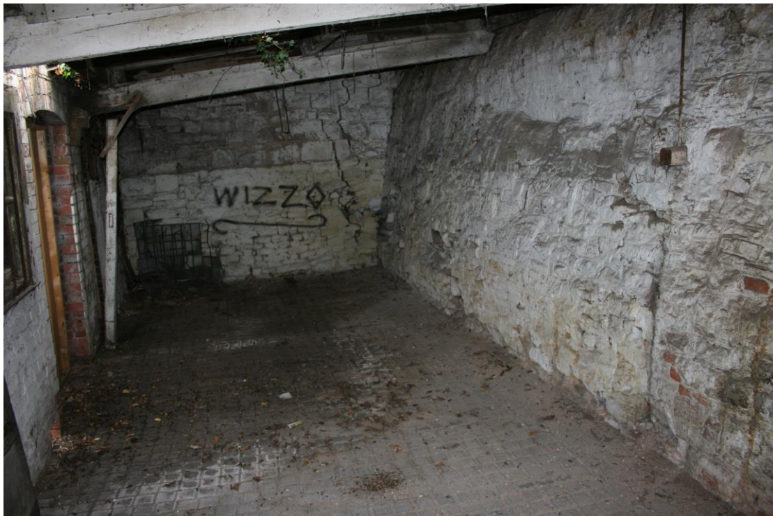
Interior (east) face of the wall in the Black Lion outbuildings
