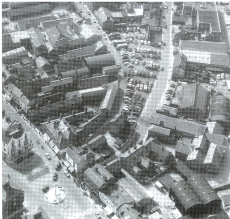
Commercial Square, shortly before the commencement of the Inner Relief Road. The site of the gate lies in front of the Kerry Arms (bottom left). From Graham Roberts The shaping of modern Hereford
