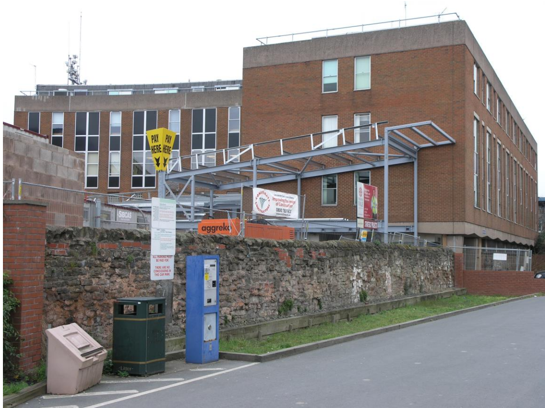
The wall and its setting to the east of the Bath Street Police Station
