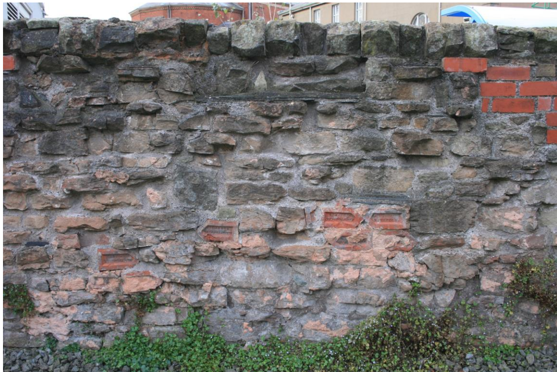
Detail of the rebuilt wall section making extensive use of 19 th -century brick at the rear of the car-park east of the Bath Street Police Station
