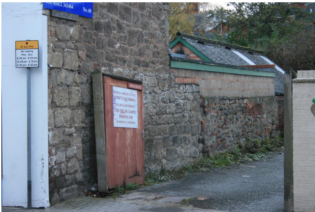
The city wall (inner face) on the south side of St Owen Street. There are clear differences between the ? primary masonry at ground-floor level, the upper floor of the frontage building, and the garden wall to the rear on the city wall line
