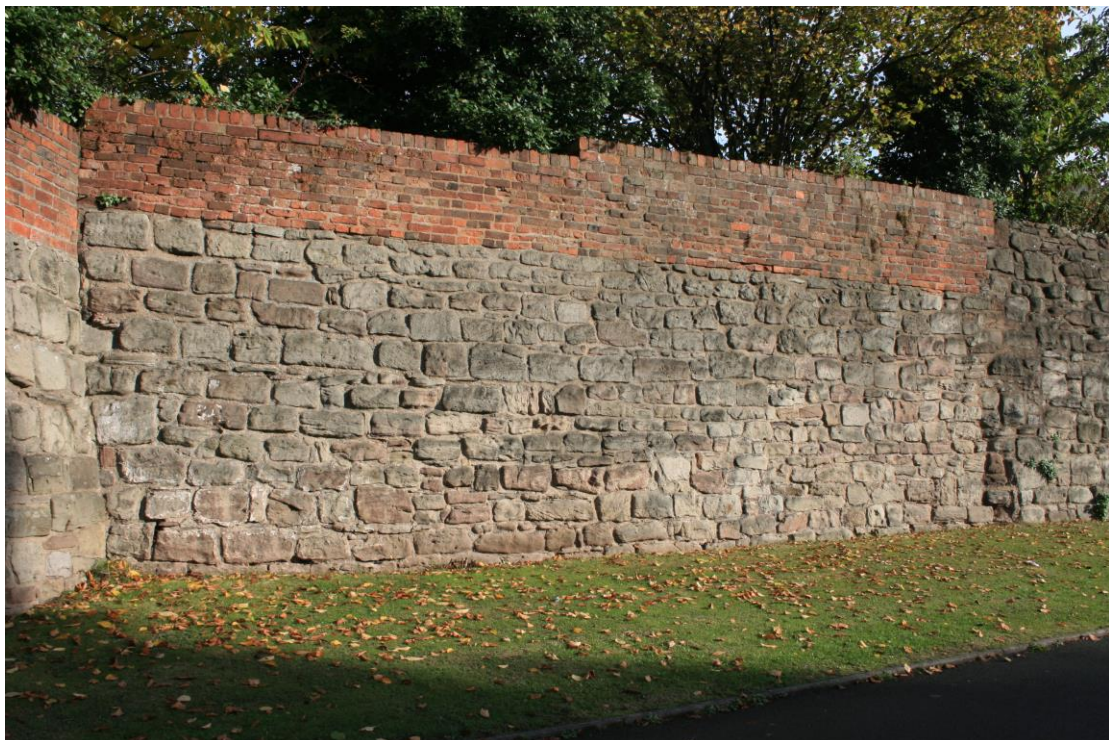
Outer face masonry of section 3 immediately south of Bastion 4
