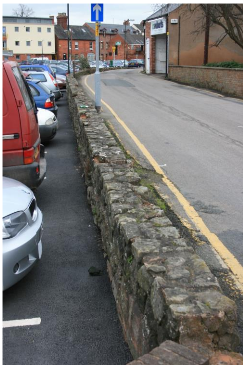
The Gaol Street/Bath Street car park wall, looking west (above), east (below). The wall beyond the lamp-post (above) is entirely modern; in front of the lamp-post the more regularly coursed masonry picks up the line of the medieval city wall. Gaol Street behind is at a higher (rampart-top) level than the car park (in the ditch)
