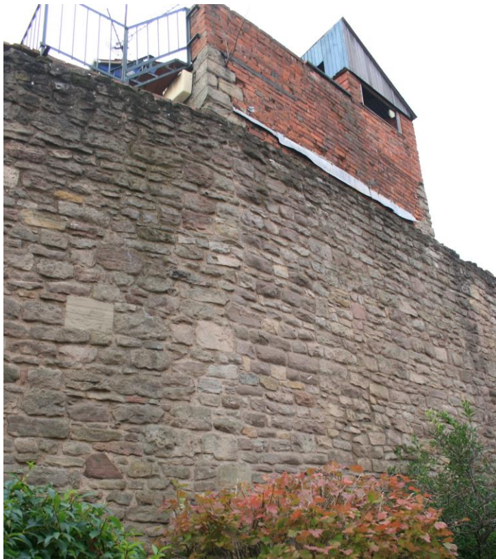
The Bastion Mews wall (exterior)
