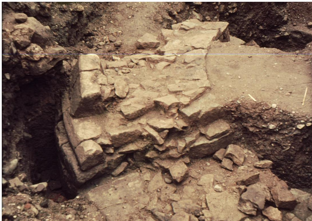
Photograph of the remains of bastion 6 under excavation in 1968; note chamfered plinth courses (for a comparison see section 16 illustrations). Photo: Ron Shoemith
