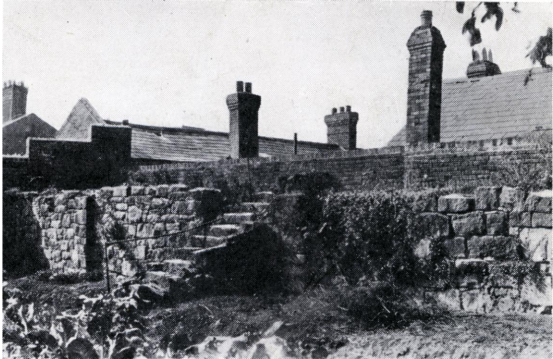
View of c.1900 probably showing buttressed interior face of the wall on the Blue Rooms nightclub plot (south of Job Centre) (courtesy Derek Foxtan)
