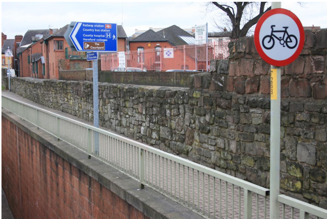
The Wall Street section, reduced in height alongside the pedestrian underpass. The eastern termination of the 1983 reproduction masonry is visible
