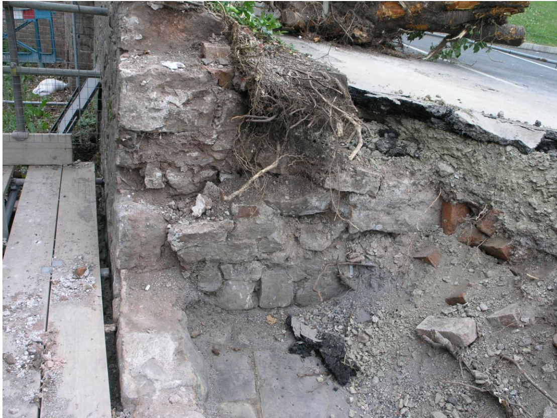
Plate 10: Masonry return and stone flagstones on line of now missing property boundary.
