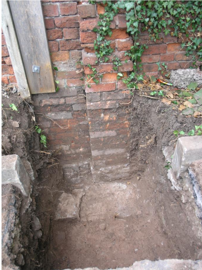
Plate 6: Looking west, showing intersection of the brick wall onto the top of the remains of the City Wall.
