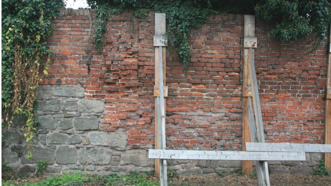
Plate 1: Northern end of the wall section: the city wall fabric is reduced in height, coinciding with a straight joint in the brickwork above. Trench 1 lies behind the wall on the left hand (northern) edge of this photo.
