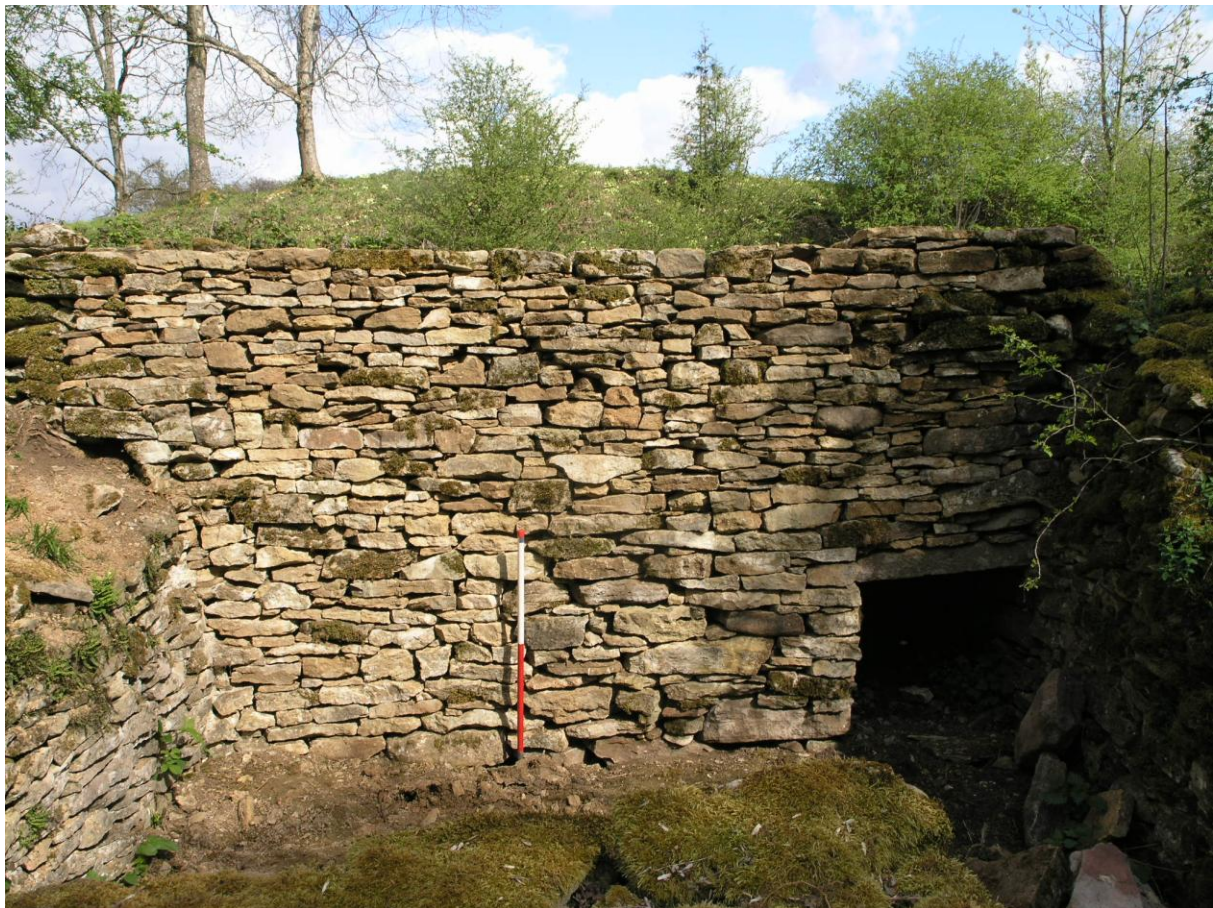
Plate 4: The northern wall after re-building
