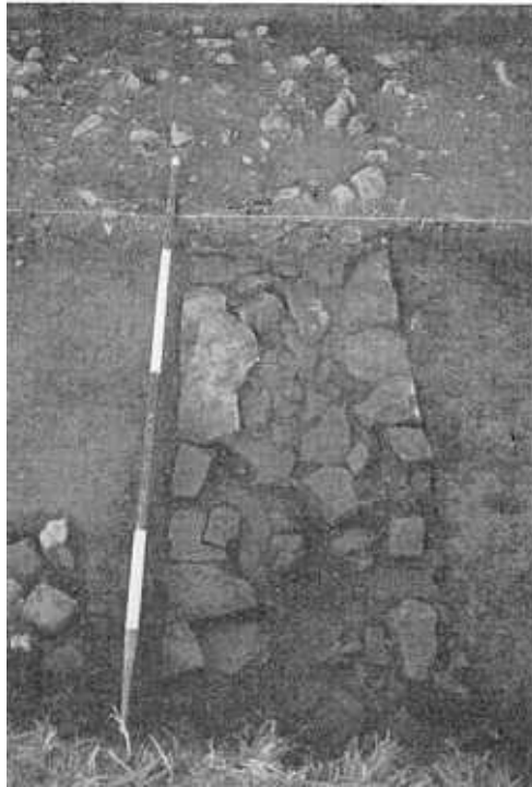
Figure 7: The top of the wall in Trench One, as revealed after removal of the superficial dumped deposit, on 12th October 1999. Viewed from the north. The scale is in divisions of 0.5 metres.
