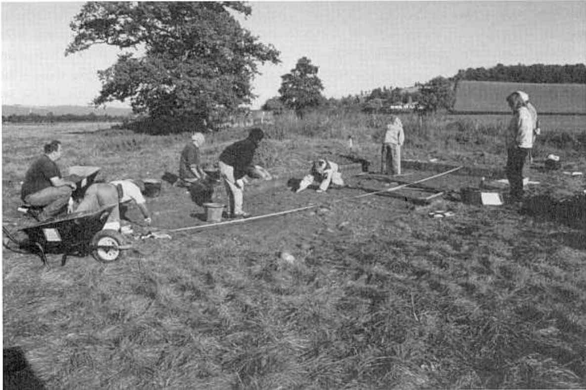
Figure 11: Trench Two from the south-east, on 12th October 1999. The rubble surface has been cleaned and is being planned.
