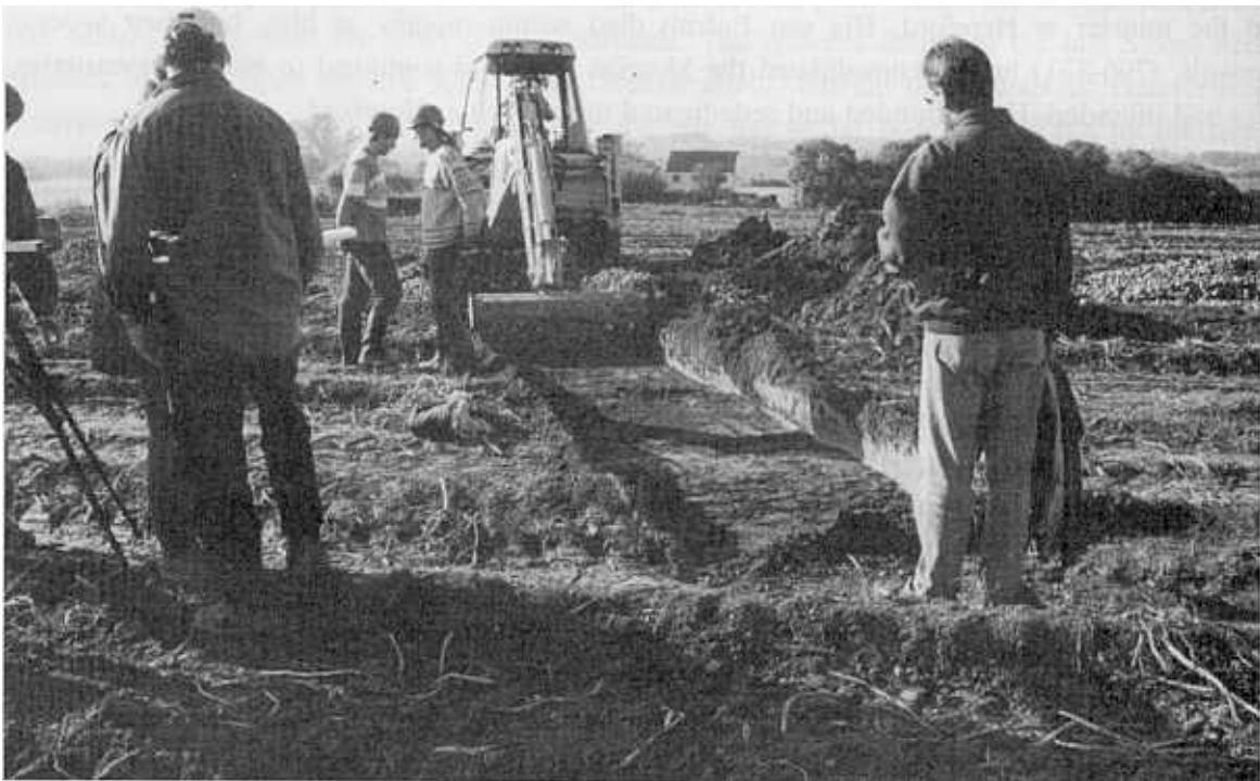
Figure 2. Initial topsoil-stripping at Trench Four (the Downfield Knoll site), 12th October 1999.
