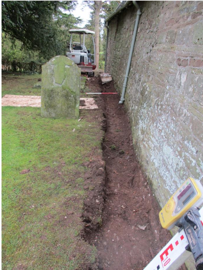
Plate 2: Drainage trench along north wall of Aylton Church, replacing concrete gutter.
