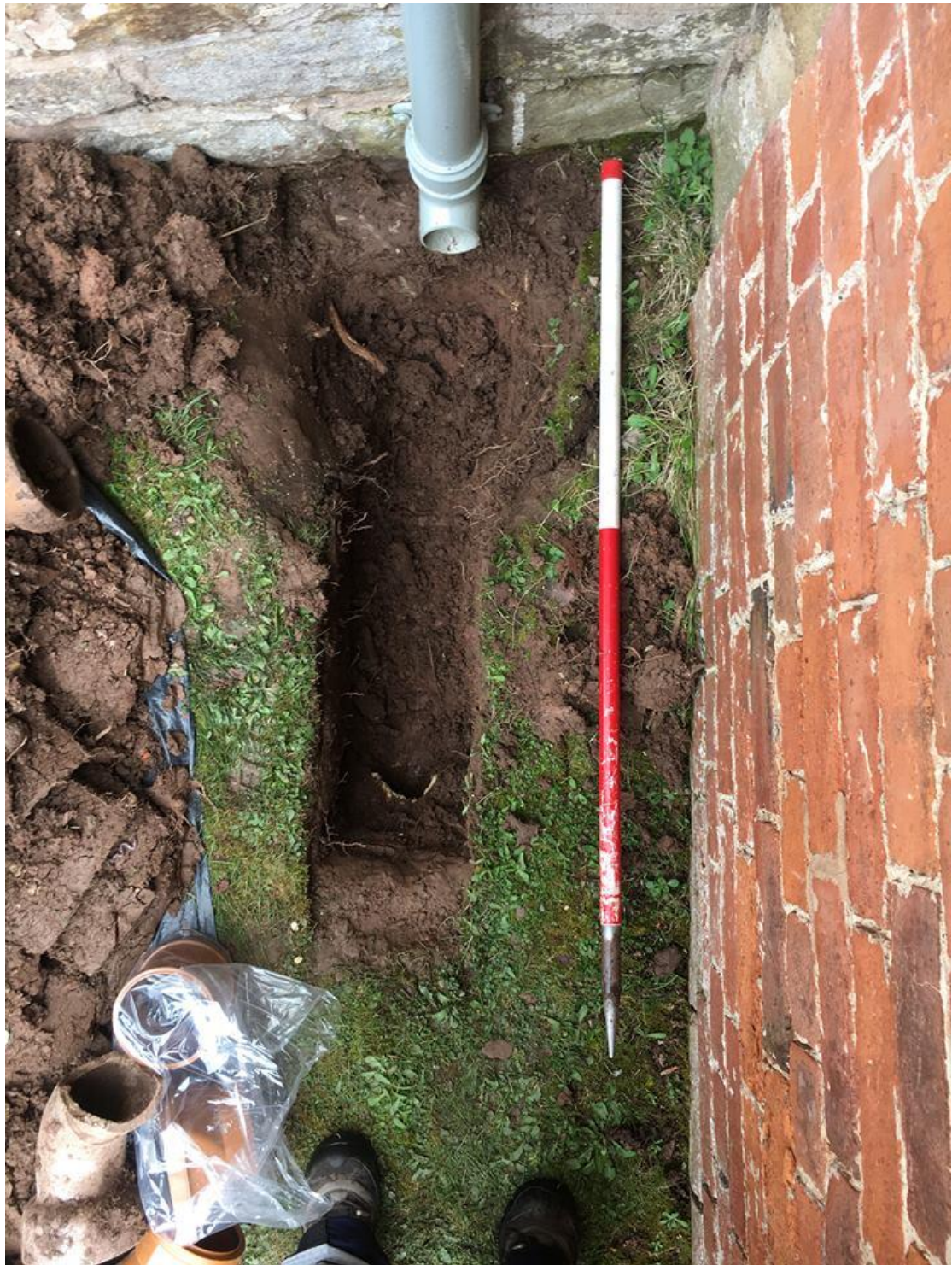
Plate 1: Trench 1 showing its location in relation to the southern wall of the church and the western wall of the porch..
