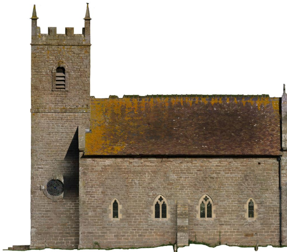
Church of the Holy Trinity, Preston Wynne, South elevation
