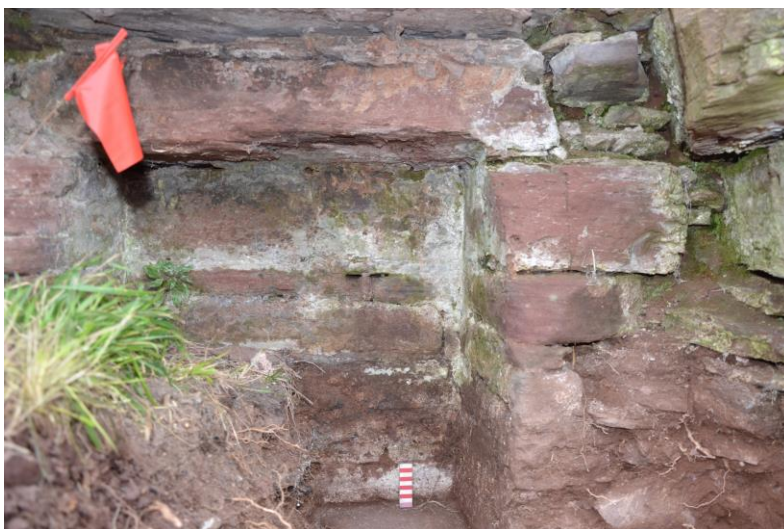
Plate 10: The partial excavation of the recess / cupboard.
