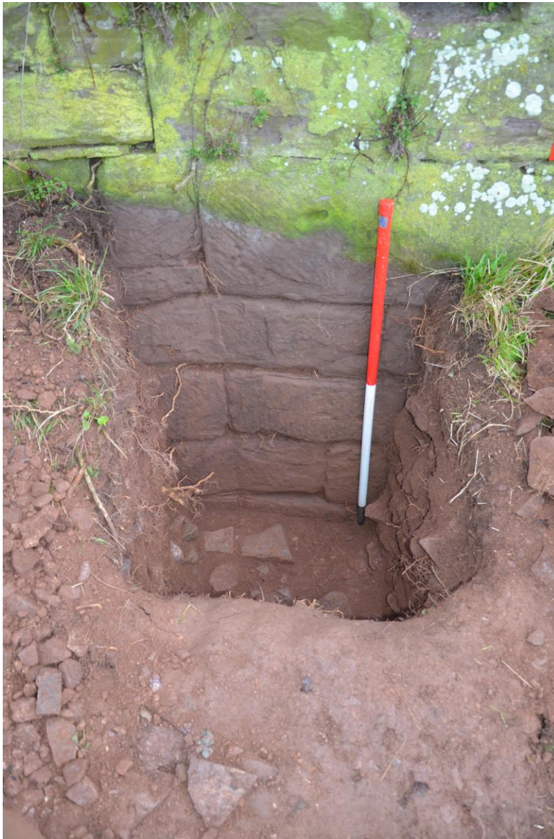
Plate 8: TP5 showing the high quality, well coursed, squared and tooled external wall facing.
