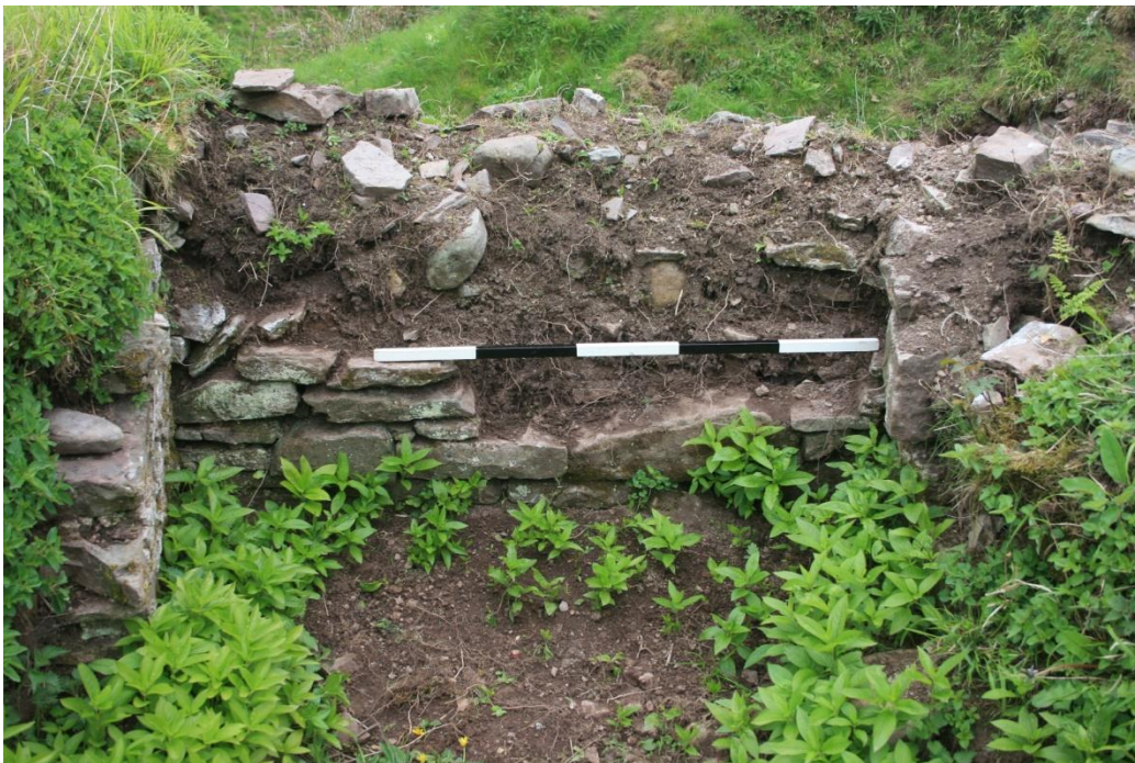
(48) NE tower, window position facing east after initial de-turfing
