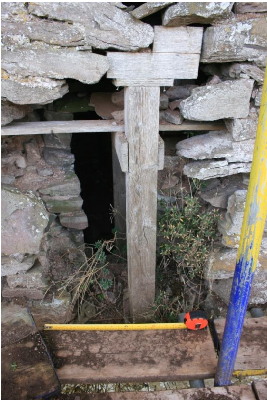
(7) Left: Damaged/propped opening into first-floor garderobe chamber. (8) Right: damaged/propped opening into first floor of tower
