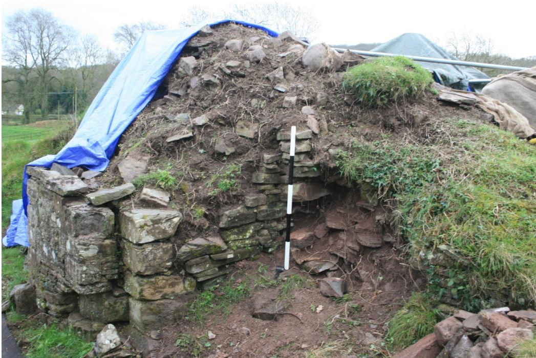
(52) Gatehouse passage, south side, inner arch before repairs
