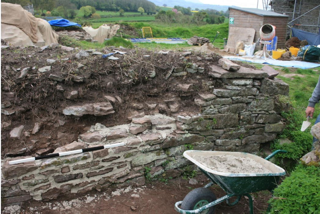
(47) N wall of gatehouse/entrance NE tower: consolidation in progress
