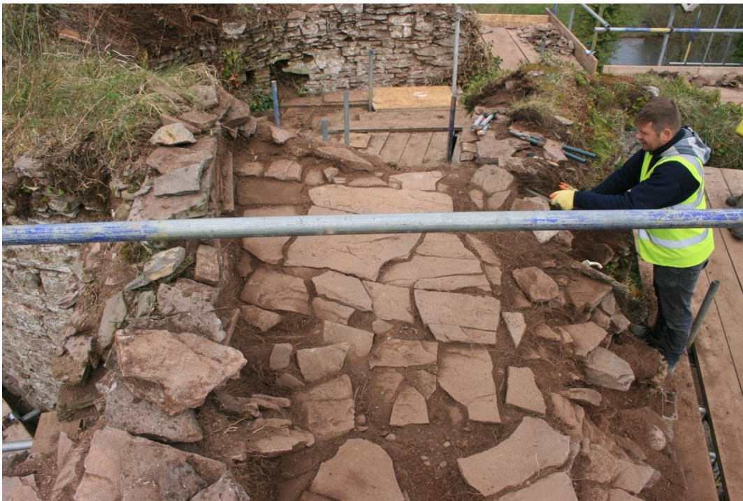
(20) Detail of wall-walk slabs at the junction with the NW tower, showing base of the one-stone thick tower wall across the line of the slabbed path.
