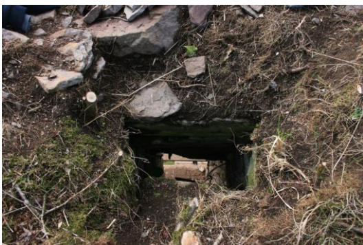
(23) The garderobe shaft open to the wall top at the S end of the west curtain, before gardening
