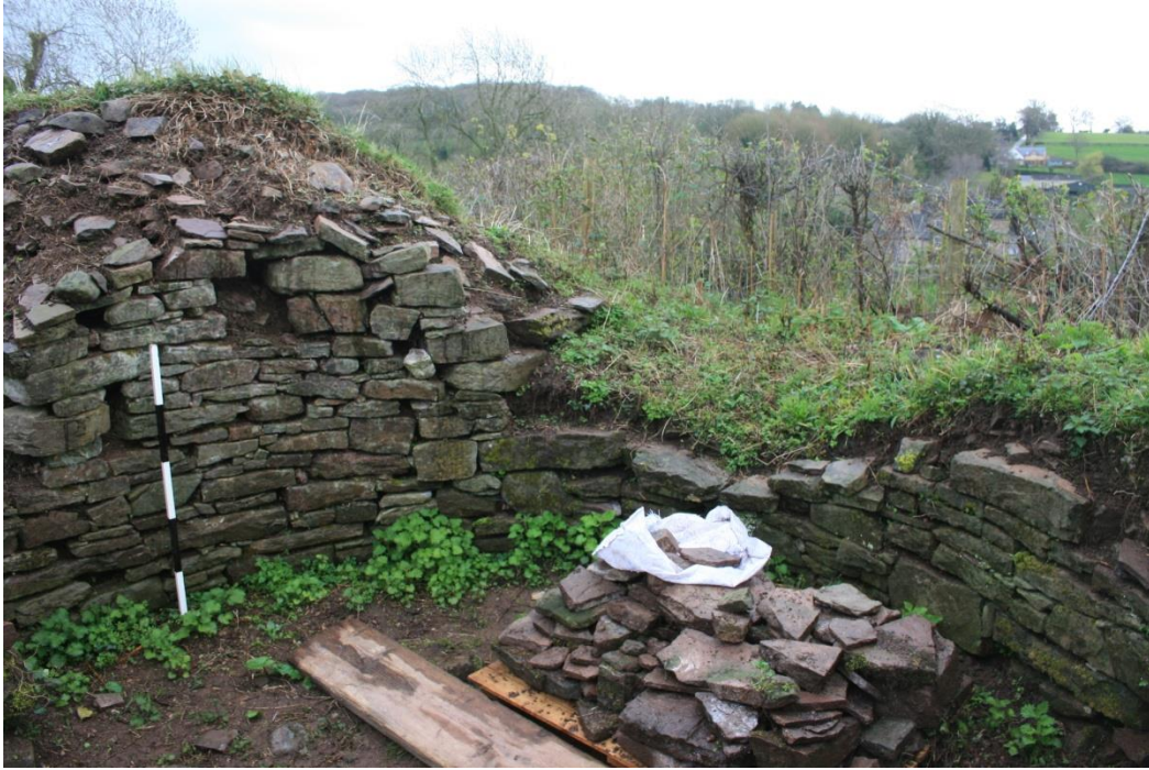
(60) SE tower, beginning of repair process, looking south
