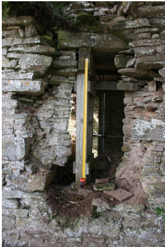
(7) Left: Damaged/propped opening into first-floor garderobe chamber. (8) Right: damaged/propped opening into first floor of tower
