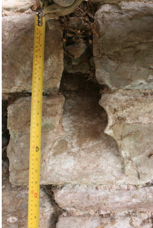
(14) Left: NW tower, first floor, loop window facing NW, detail of eroded loop terminal and its blocking; (15) Right: NW tower, first floor loop window, detail of loop terminal
