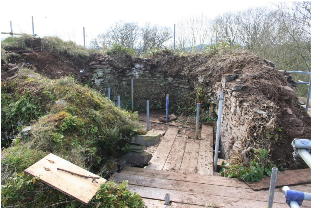
(18) NW tower wall tops, at an early stage of gardening, looking west through the gap in the wall over the first-floor doorway into the hall
