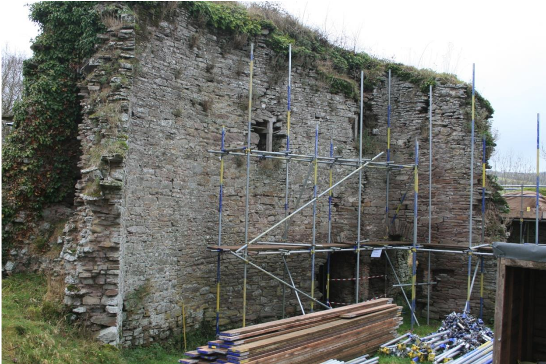
(3) The west curtain wall, looking NW, before repairs
