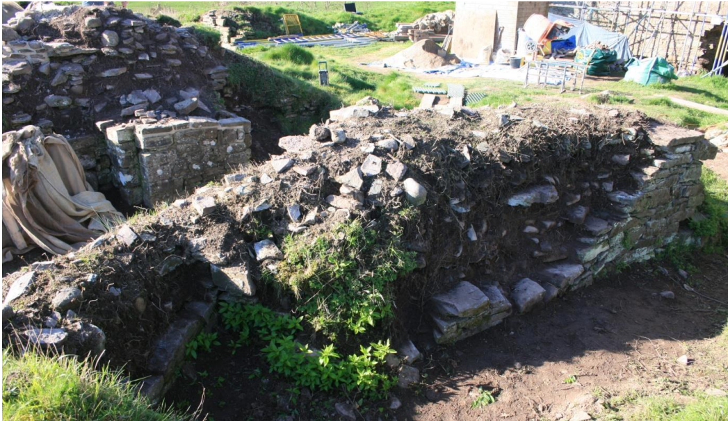
(46) N wall of gatehouse passage/S wall of NE tower, commencement of gardening process showing limits of survival of facing stones in entrance to NE tower
