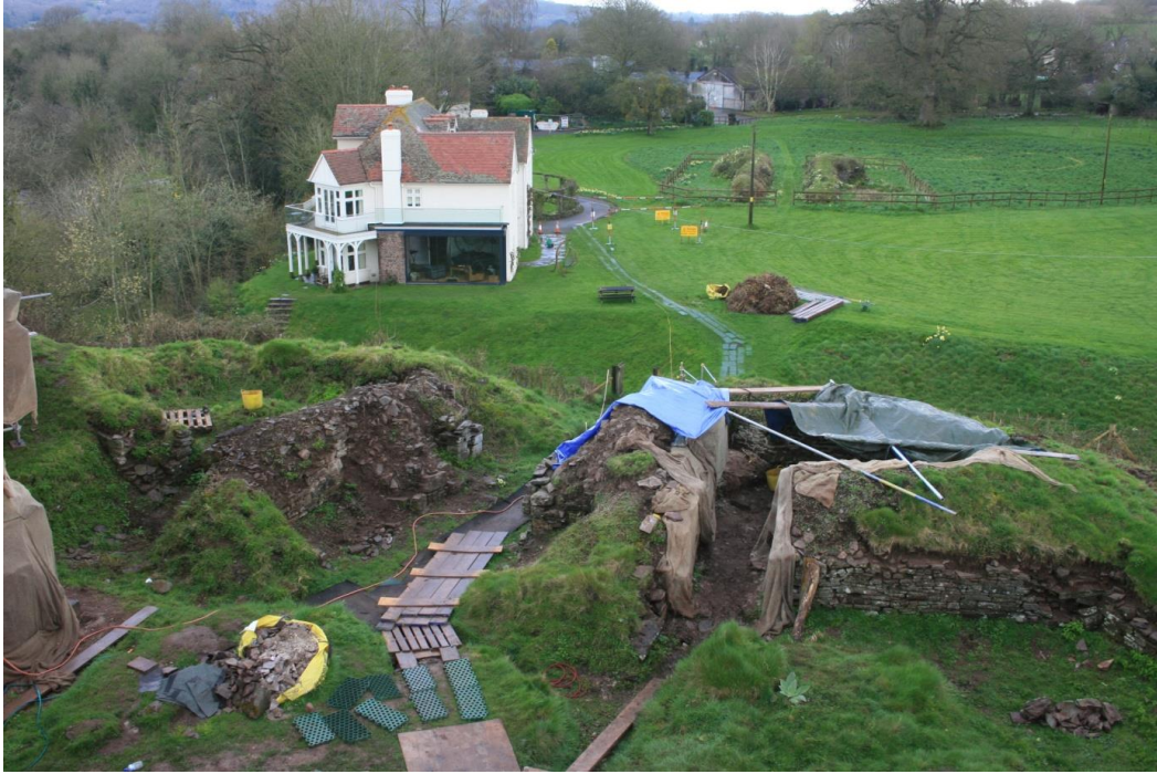
(45) General view looking east towards the outer bailey during gatehouse repairs
