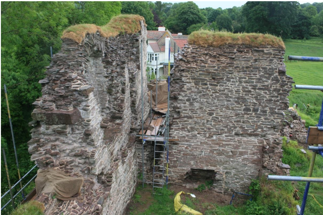
(40) The north and east walls of the hall, post-repair; note fireplace position at near end of north wall (bottom left), doorway through end wall into chamber beyond and (consolidated) cupboard/niche opening in centre of wall
