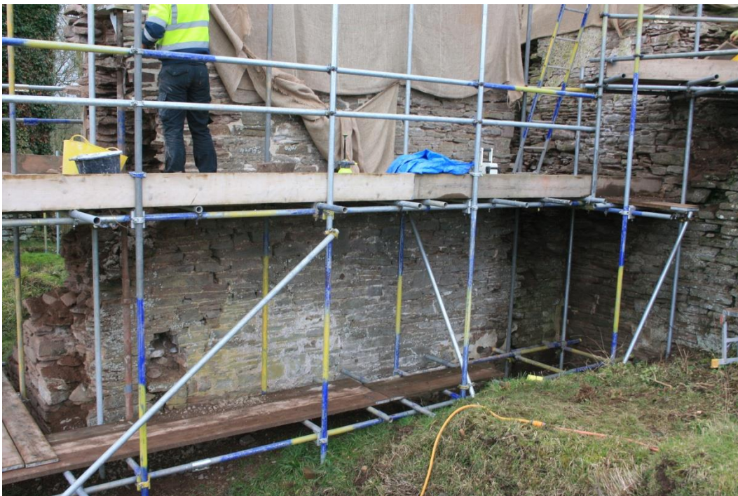
(42) E end wall of hall, external, during re-pointing
