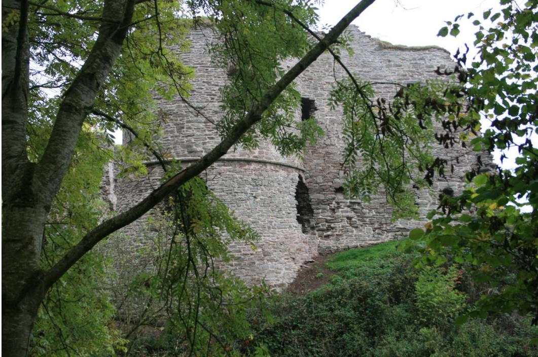
(11) General view of west elevation, looking south-east from the Hornwork, post-repair
