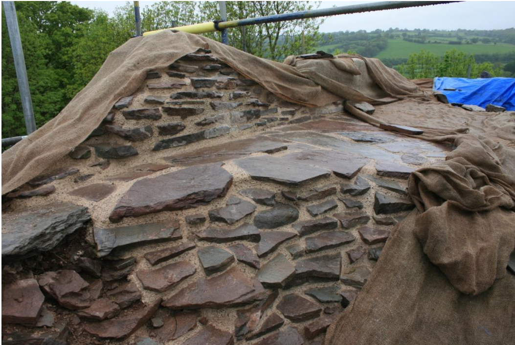
(24) The parapet wall and wall-walk as consolidated prior to soft capping
