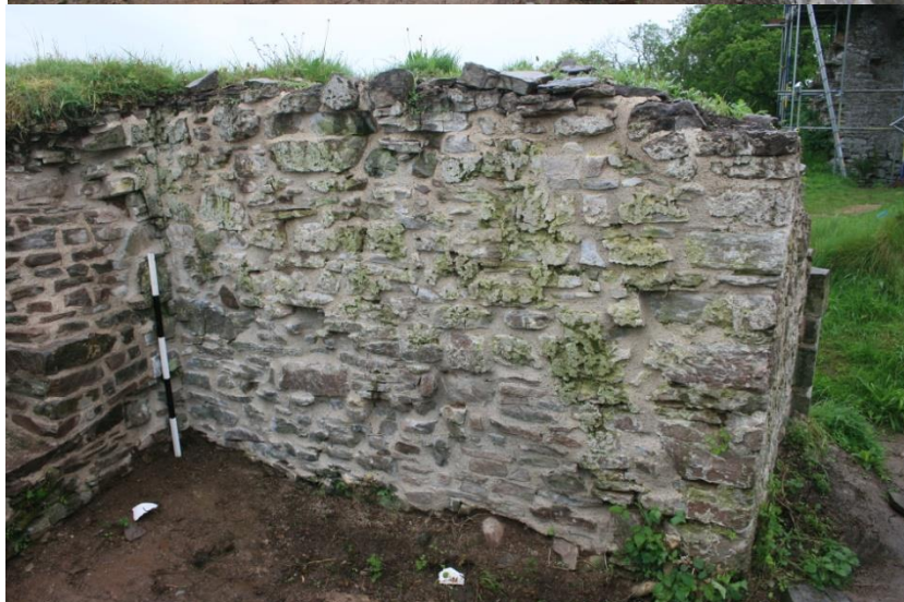
East tower interior after repair: (55) top, north side and NE-facing window position; (56) middle, SE facing window position; (57) bottom, west wall (with partly surviving render) and doorway to courtyard
