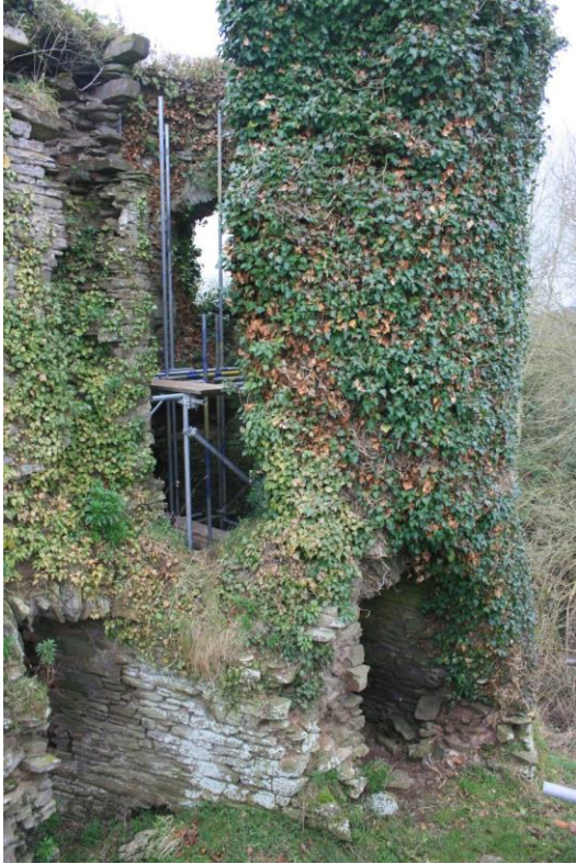
(33) Left: SE side of the NW tower showing first-floor doorway to hall with damage above and to its left, passage below and N-facing window embrasure in tower base; (34) Right: S side of doorway from tower first-floor chamber
