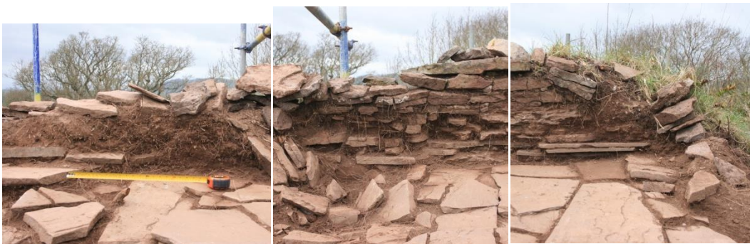
(22) Composite photo of inside (east) face of the parapet wall, as first exposed, with S wall of tower extreme right, damaged area to slabbed surface centre
