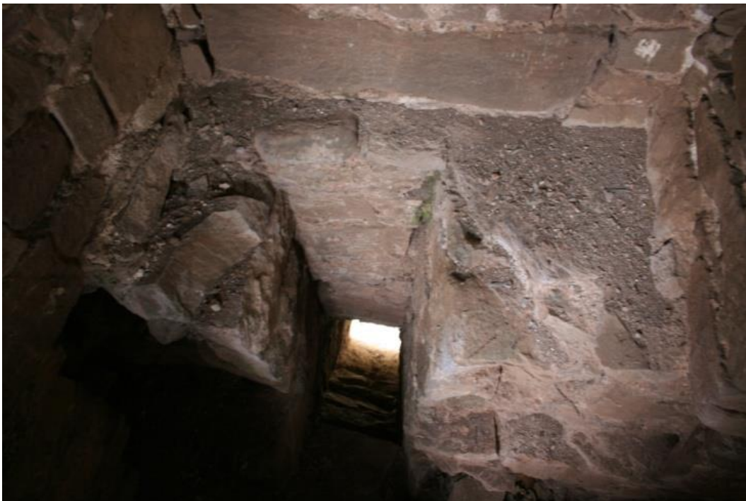
(10) Looking down main garderobe chute from seat position to outlet in west wall face
