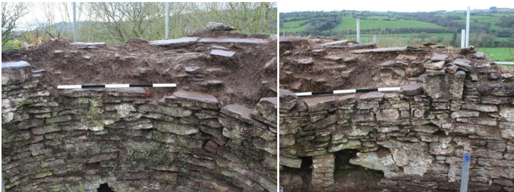
(27) NW tower wall top, W and NW sides
