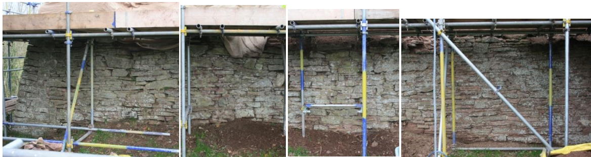
(37) North wall, pre-repair composite photo of undercroft level masonry
