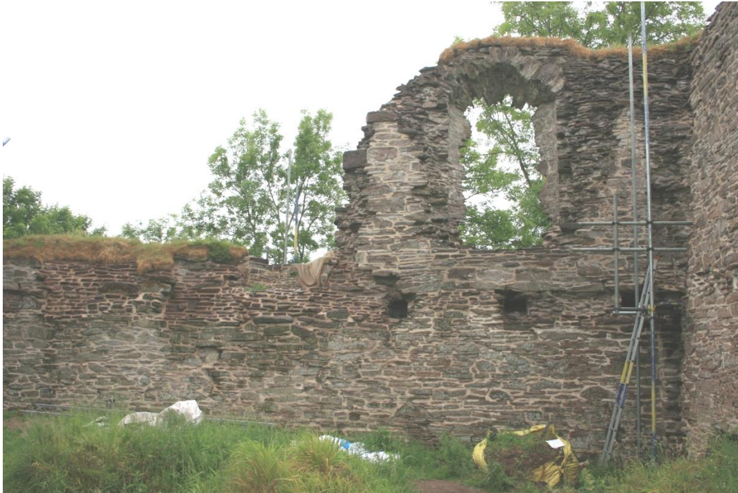
(36) North wall, internal elevation of eastern half, post-repair
