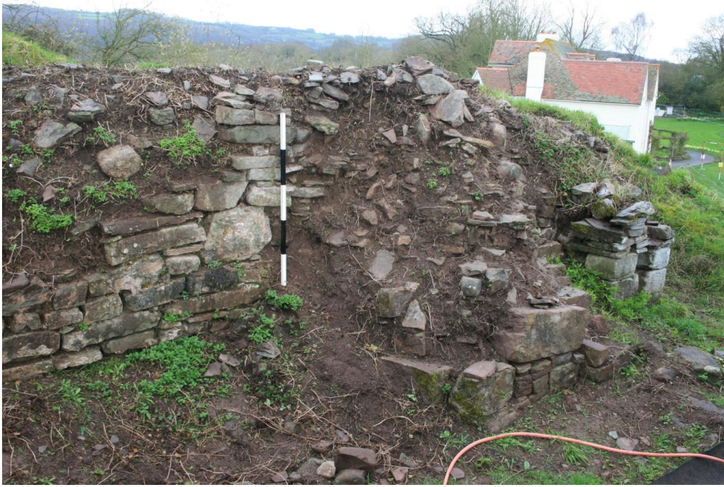
(49) Gatehouse entrance passage, north side, inner arch, before repair
