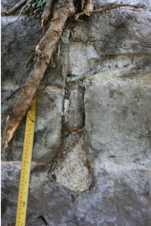
(14) Left: NW tower, first floor, loop window facing NW, detail of eroded loop terminal and its blocking; (15) Right: NW tower, first floor loop window, detail of loop terminal
