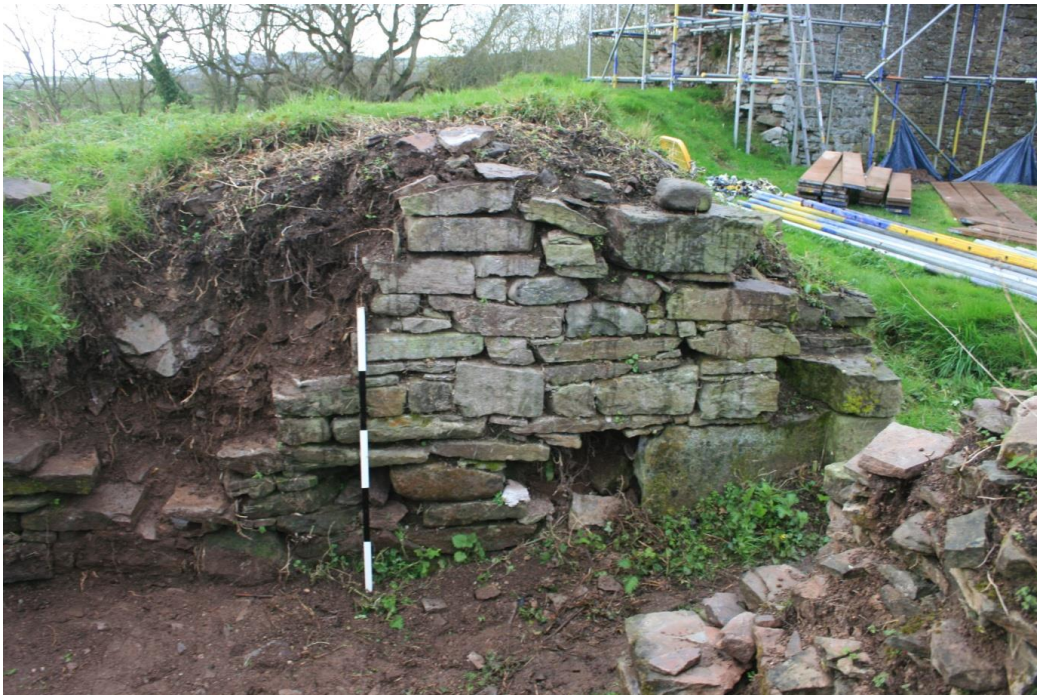
(61) SE tower, beginning of repairs, west wall and courtyard doorway
