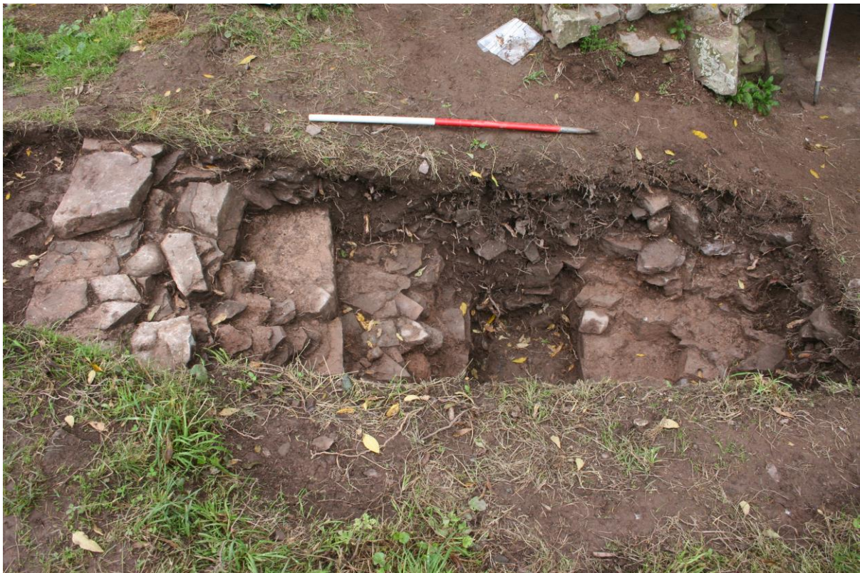
Test Pit 1, looking south. The left-hand wall with footings on three levels is the end wall of the hall/chamber-block undercroft; the right-hand wall is the original exterior end wall of the hall/chamber block, joining the fabric of the NW tower (top right corner)
