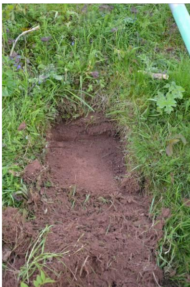
Plate 22: Detail showing depth of sole plate excavations for scaffold construction.
