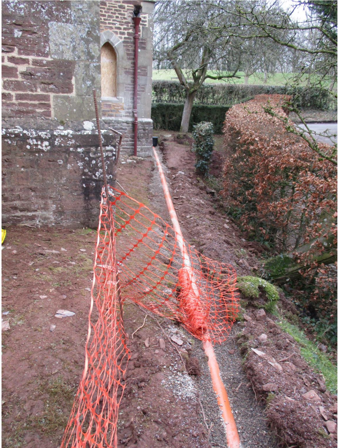
Plate 1: Drainage run looking north.
