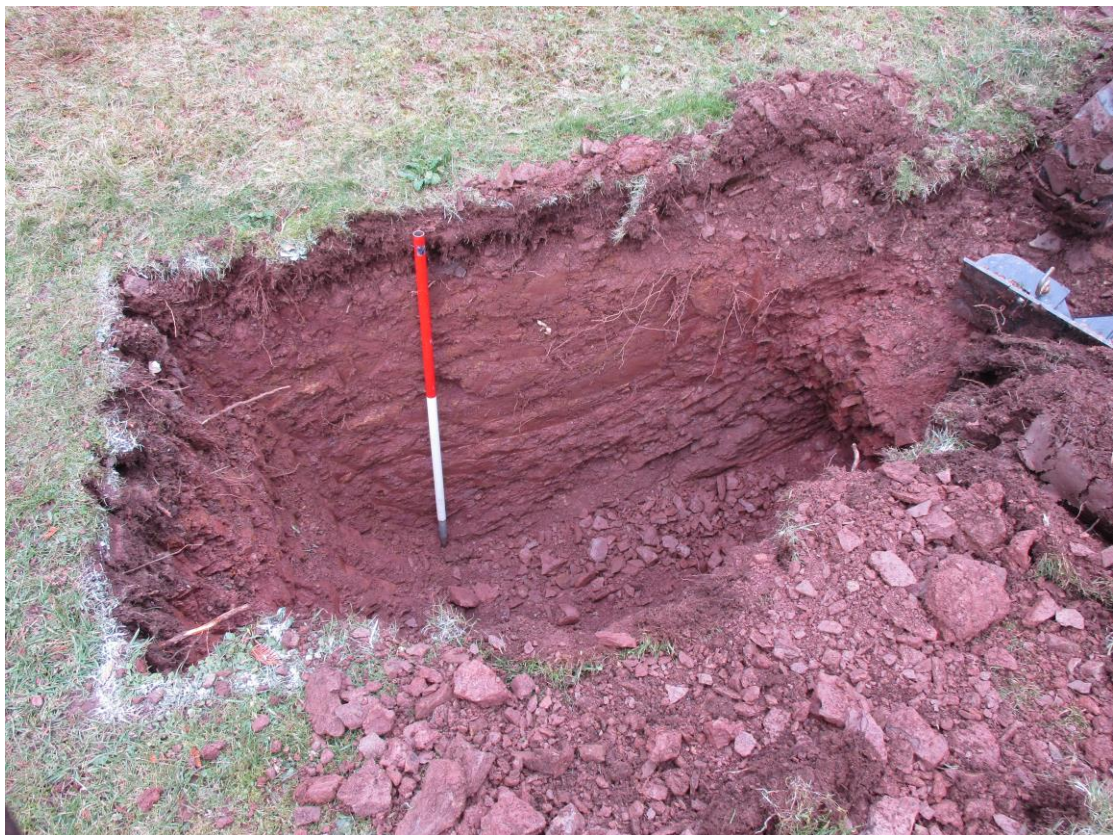
Plate 4: Trench for soakaway
