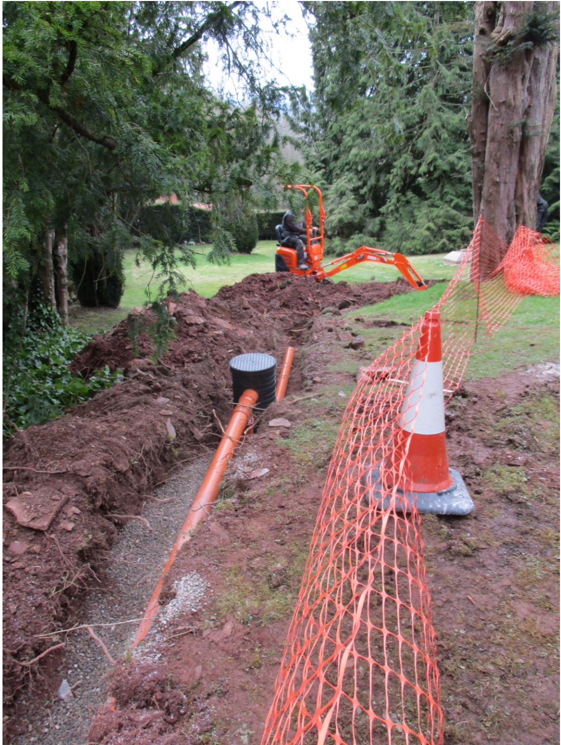
Plate 2: Drainage run looking south
