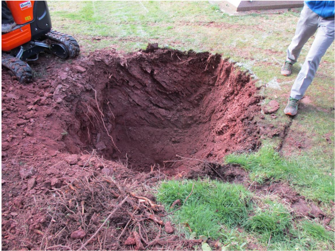
Plate 3: trench for sewage treatment plant.
