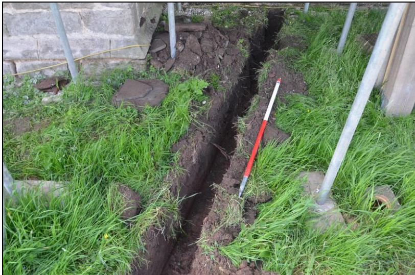
Plate 3: facing south, overview showing excavation of the Service trench.
