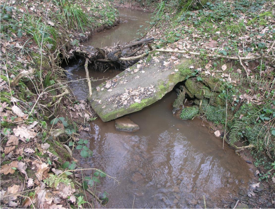
Figure 9: Stone foot bridge (HSM 76756)
