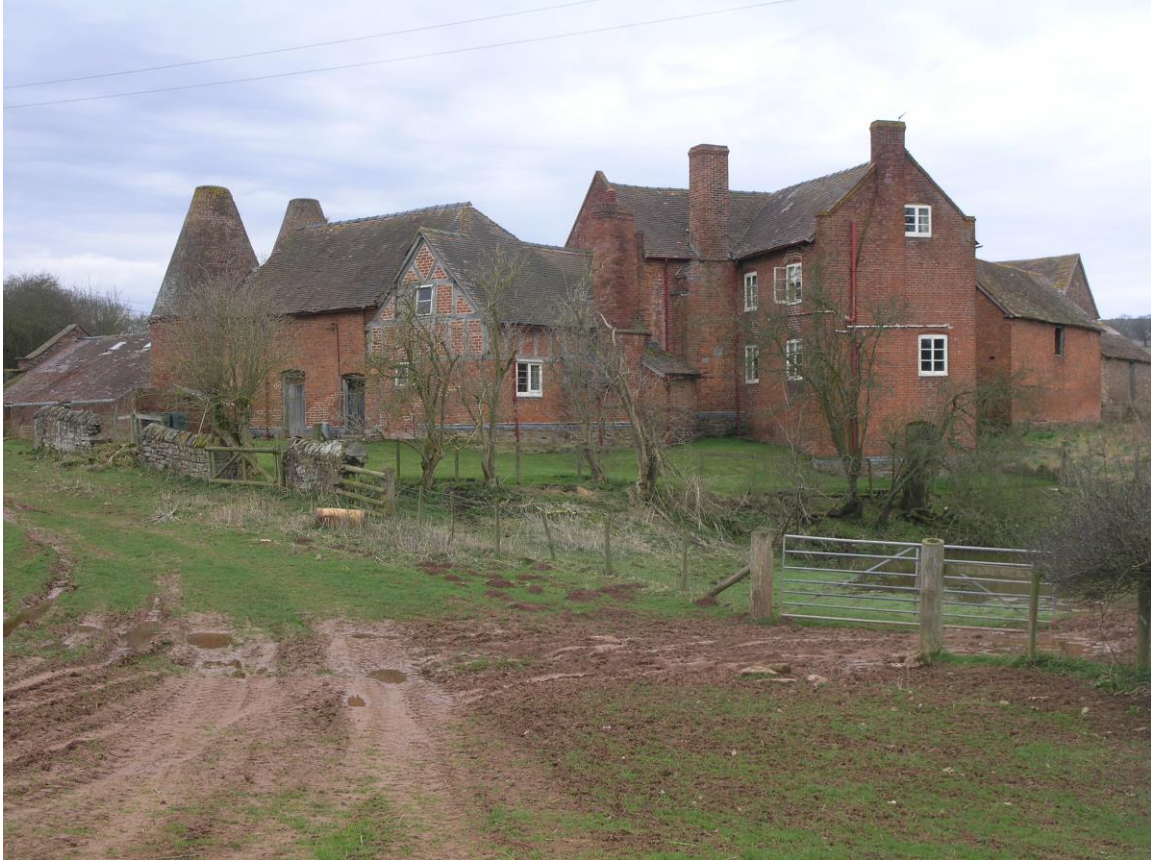
Figure 12: The complex of buildings known as “The Farm”.
