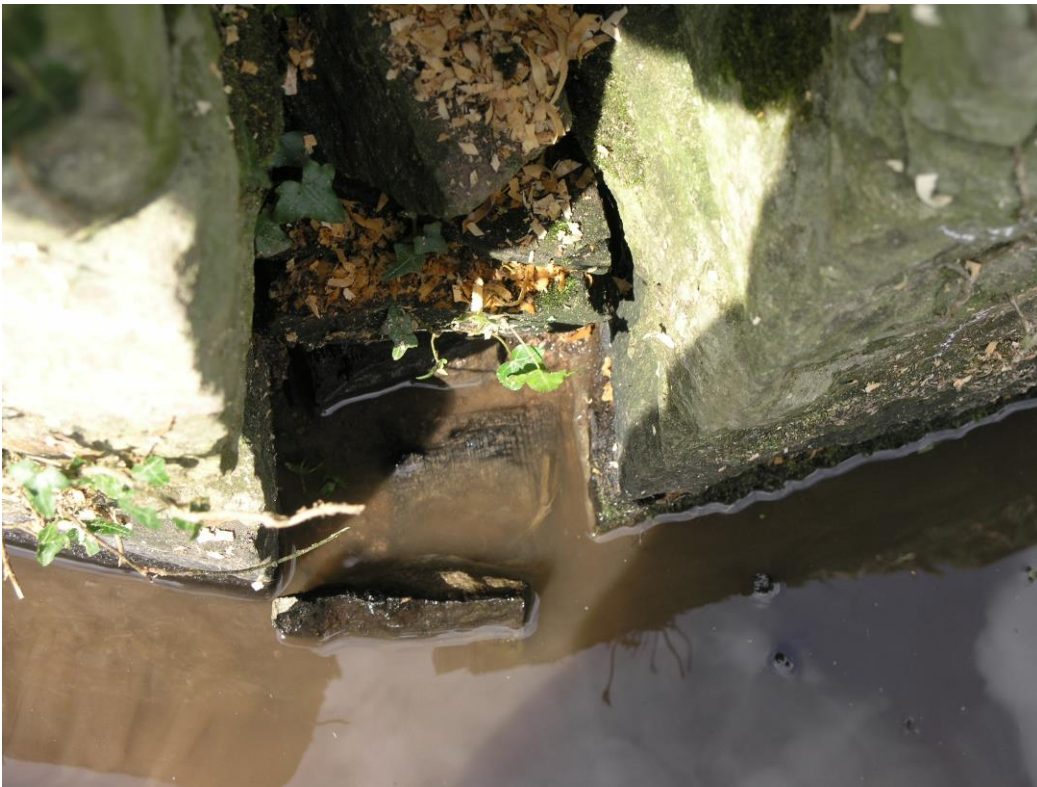
Plate 8: Detail of recess in Western Elevation showing remains of timber post.
