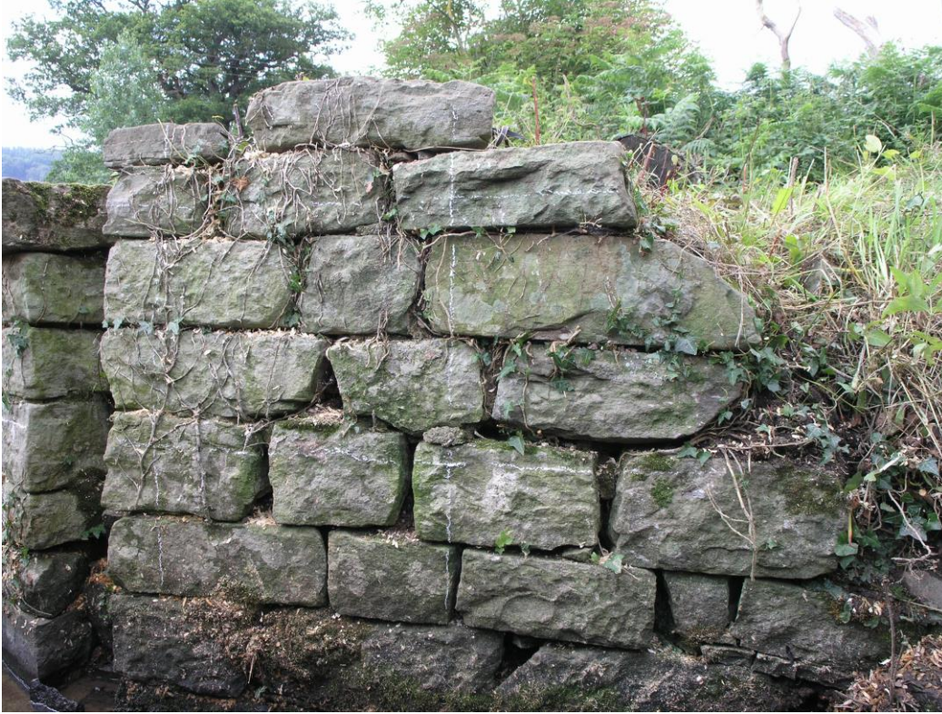
Plate 3: Western elevation, face A
