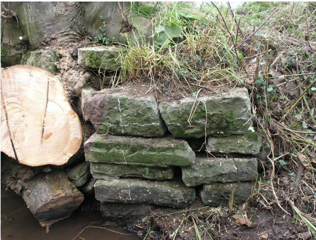
Plate 6: Eastern Elevation, Face D
