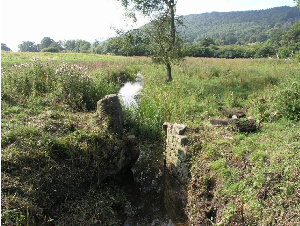
Plate 1: General view of sluice looking south
