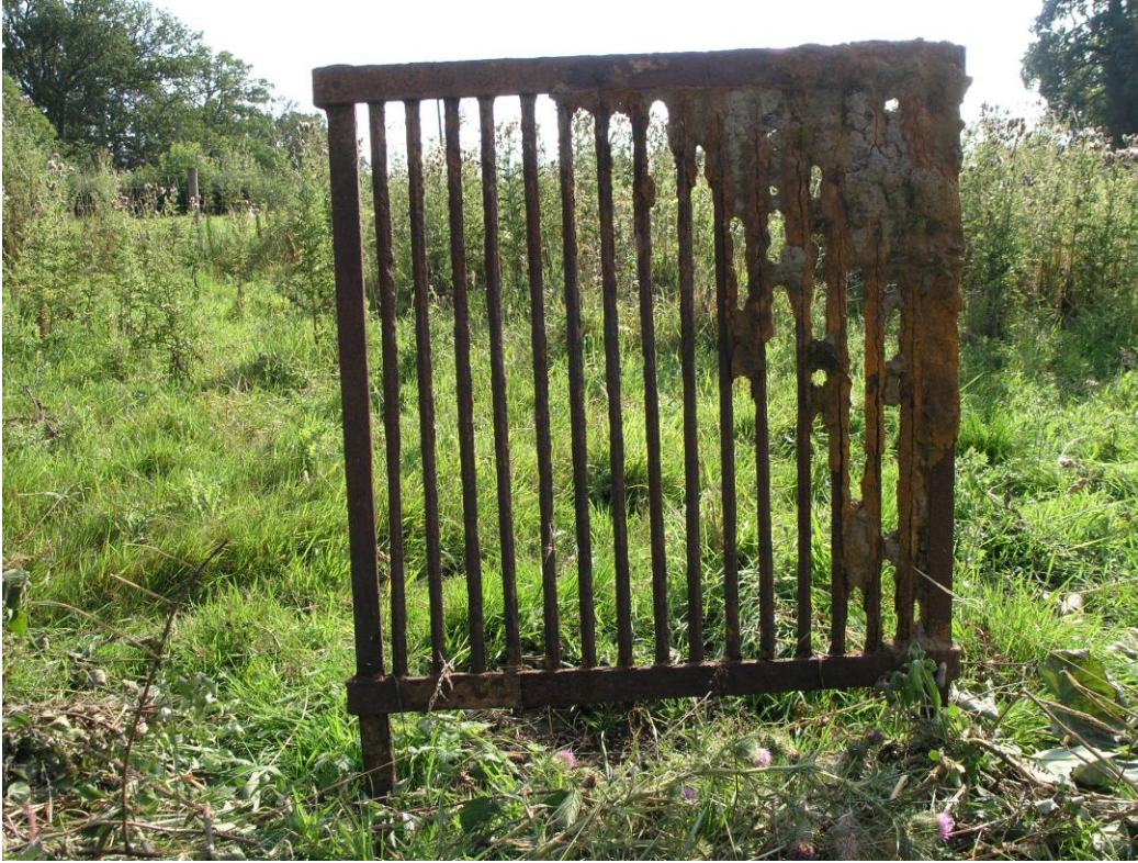
Plate 11: Iron grille originally located at mouth of culvert.
