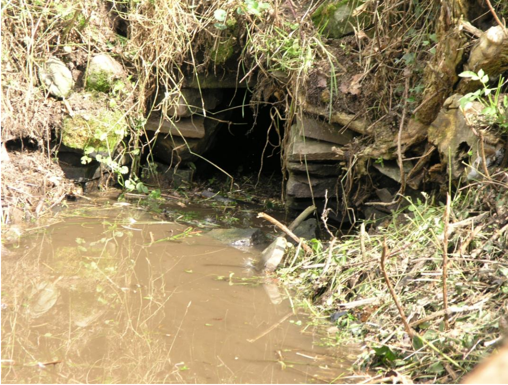
Plate 9: Culvert looking North,
