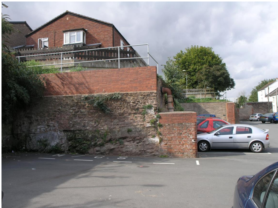
Fig 24 Terracing (part built, part cut bedrock) on the south side of Kyrle Street on the site of the 19 th -century gasworks
