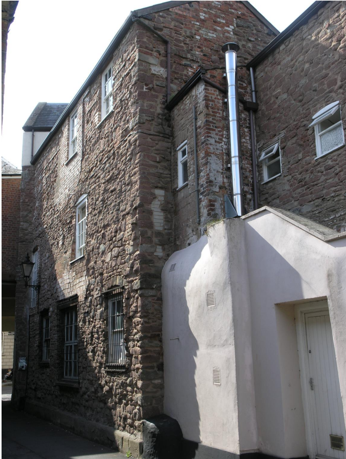
Fig.8 6 High Street: side/rear view, from entry. Assumed to be early 19 th -century
