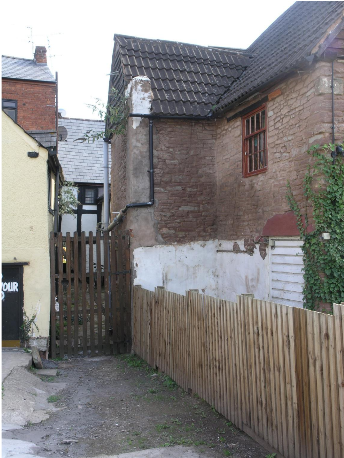
Fig.6 Rear view of passage between 1 Brookend Street and 30-32 Broad Street with timber framing and sandstone rear wing
