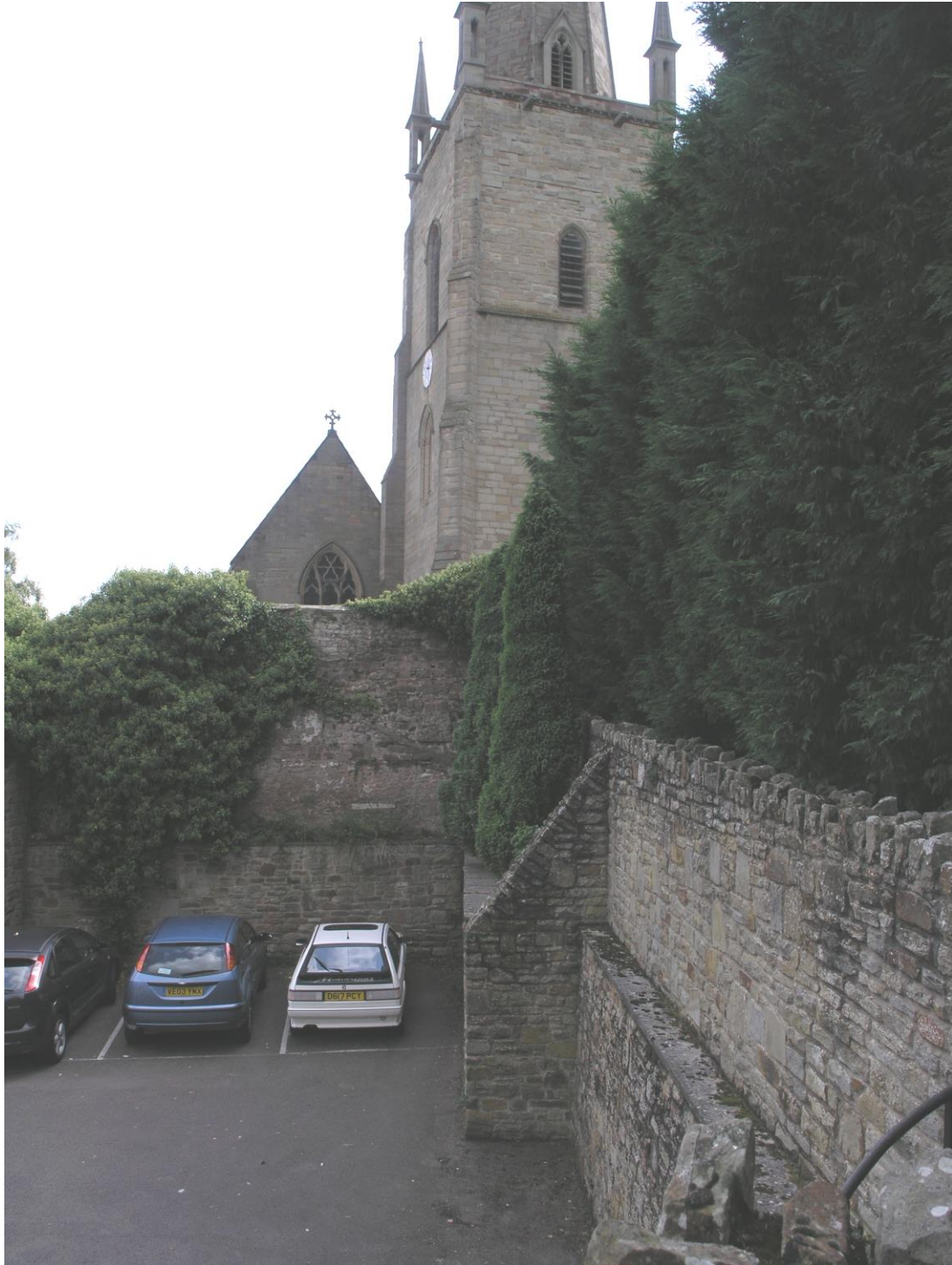
Fig. 16 The courtyard/car-park of the Royal Hotel, deeply terraced into the rising ground towards St Mary's Church
