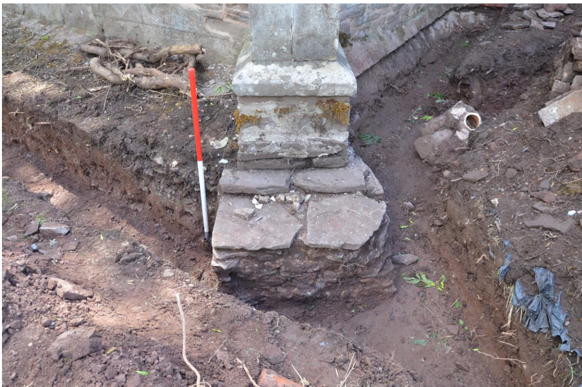
Plate 2: Detail of foundations for the north-western corner buttress for the chancel.
