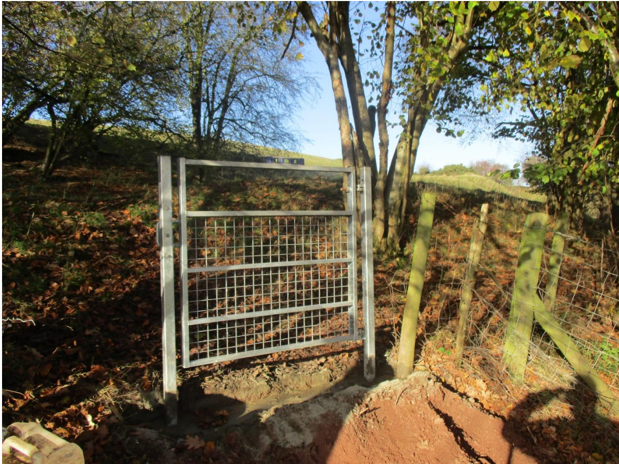
Plate 2: The replacement gate after concreting.
