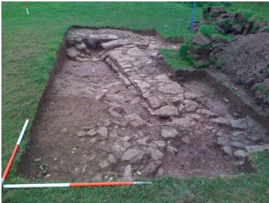
Figure 23: Medieval wall foundation [224], the rubble layer in the foreground, left of the wall is the fill [225] within construction trench (226). © Chris Atkinson
