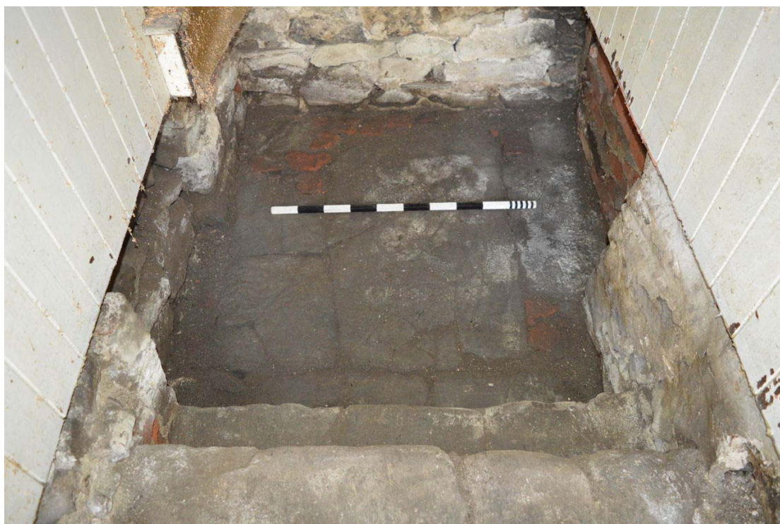
Fig. 7 The stone steps and flag stone floor revealed beneath the suspended floor, viewed from the north-east. Note the blocked doorways to left and right. Photo CPAT 3888-0006
