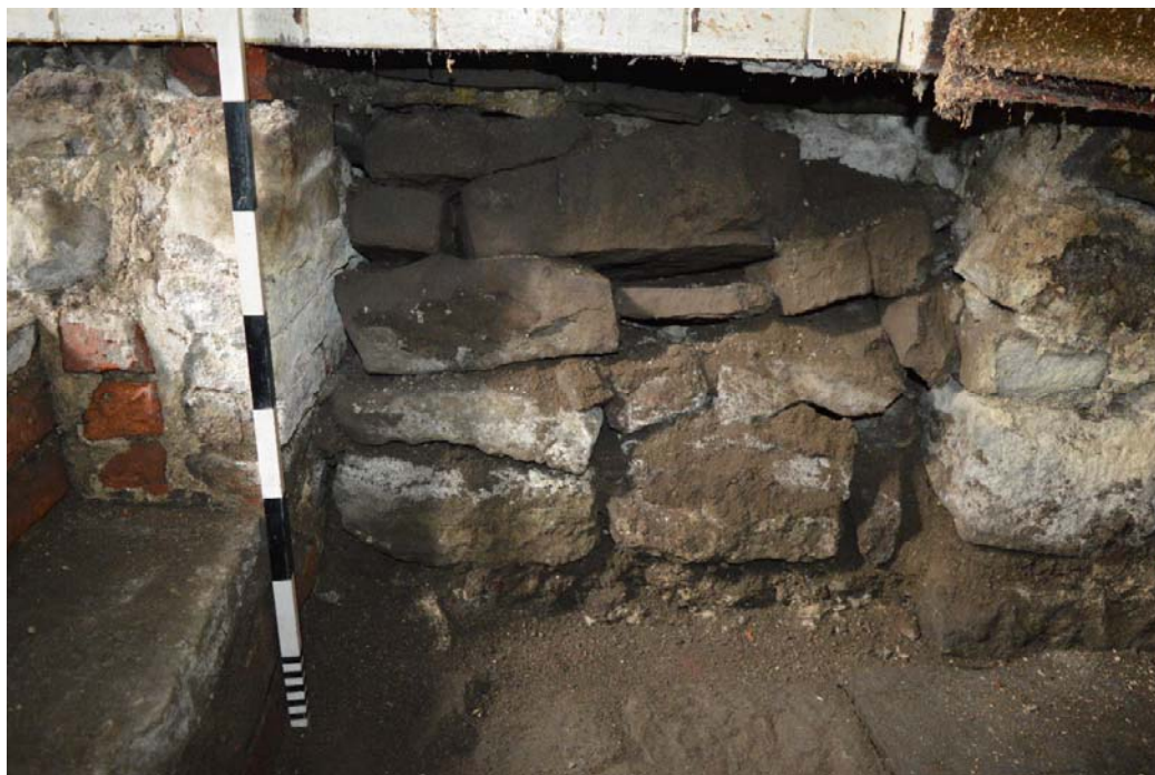
Fig. 8 The blocked entrance, viewed from the north-west. Photo CPAT 3888-0010
