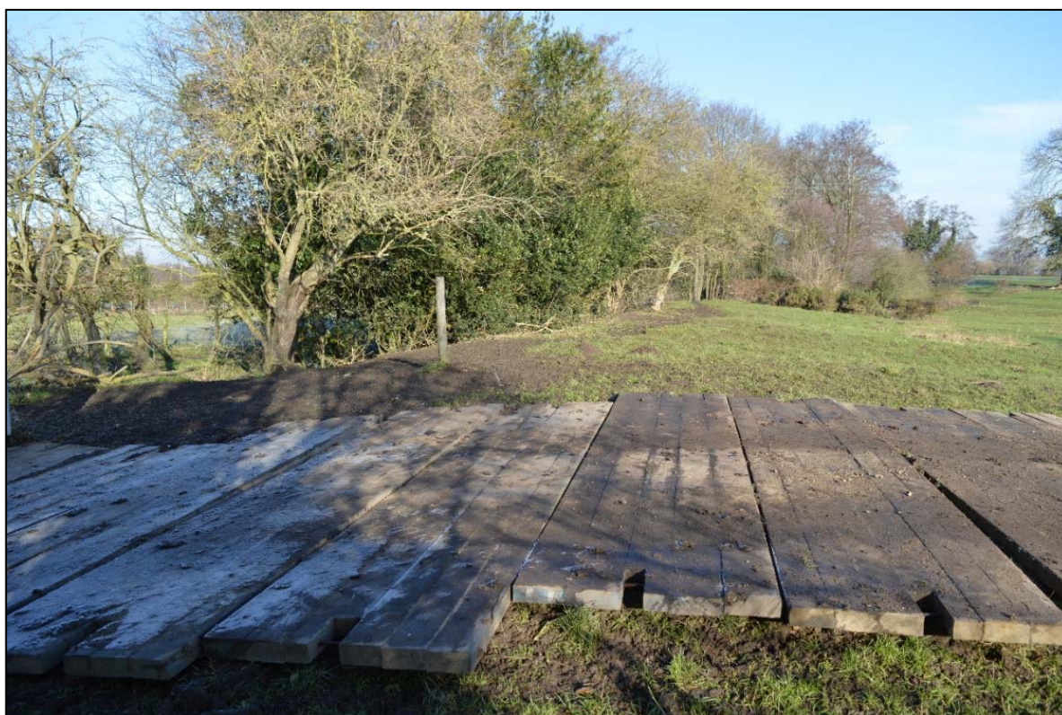
Fig. 2. The bog matting laid over the access track crossing Wat's Dyke (SAM De154) south of Black Brook Bridge (CPAT Photo 3904-0016).
