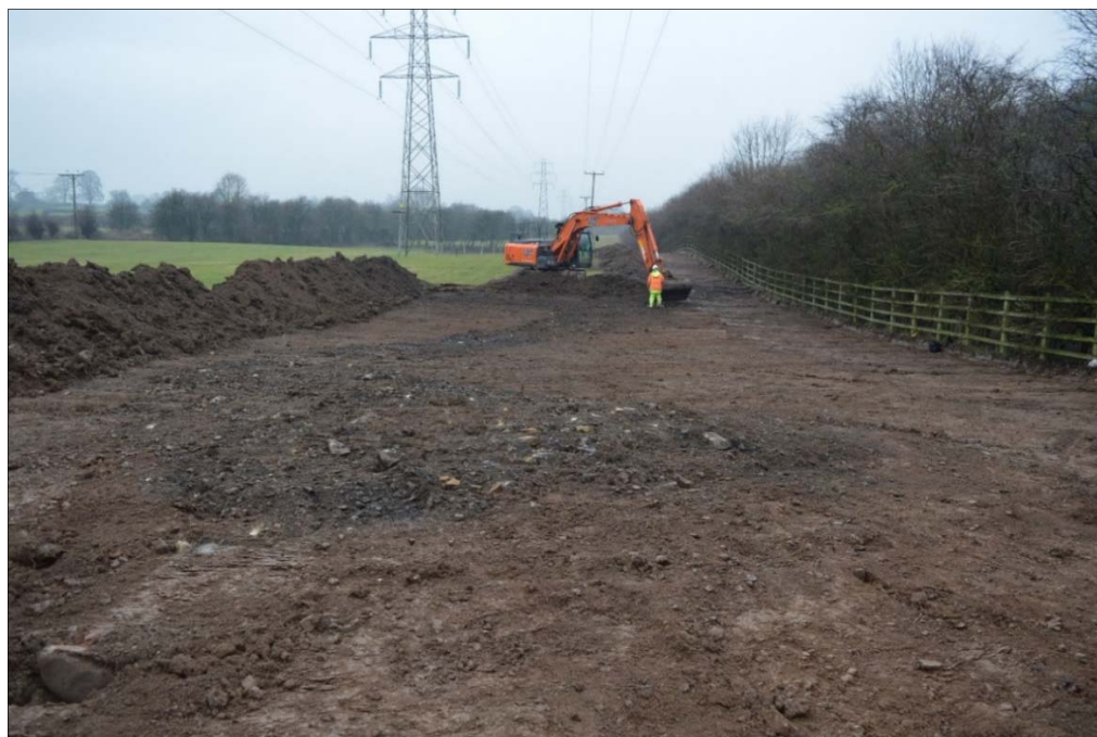
Figure 8. Trackway viewed from the south © CPAT 3958-0076
