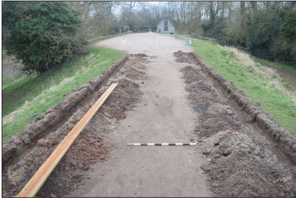
Fig. 6 Groundworks on the dam/tiltyard viewed from the north Photo CPAT 4915-017
