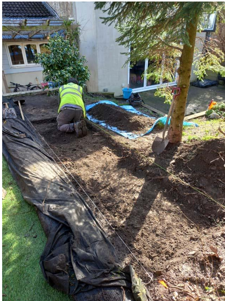
Fig. 3 Excavation to base of topsoil context (001) looking south-east. Photo CPAT 4975-011
