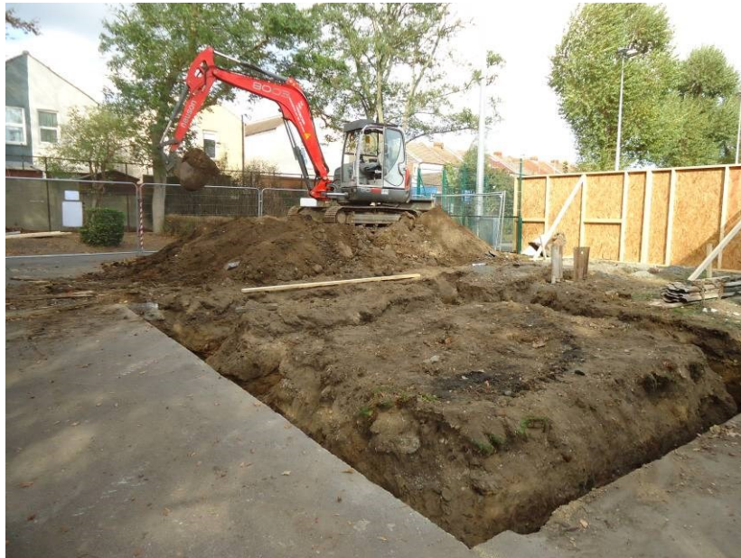
Fig 3: View of the site and trenches.
