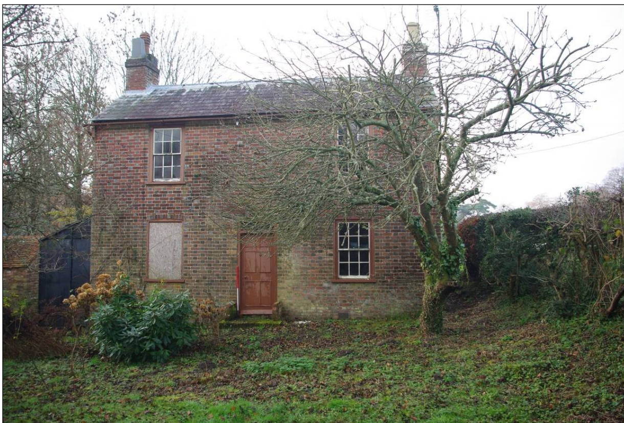
Figure 2. East elevation (front). Note possibly original slate chimney pot on right hand stack.
