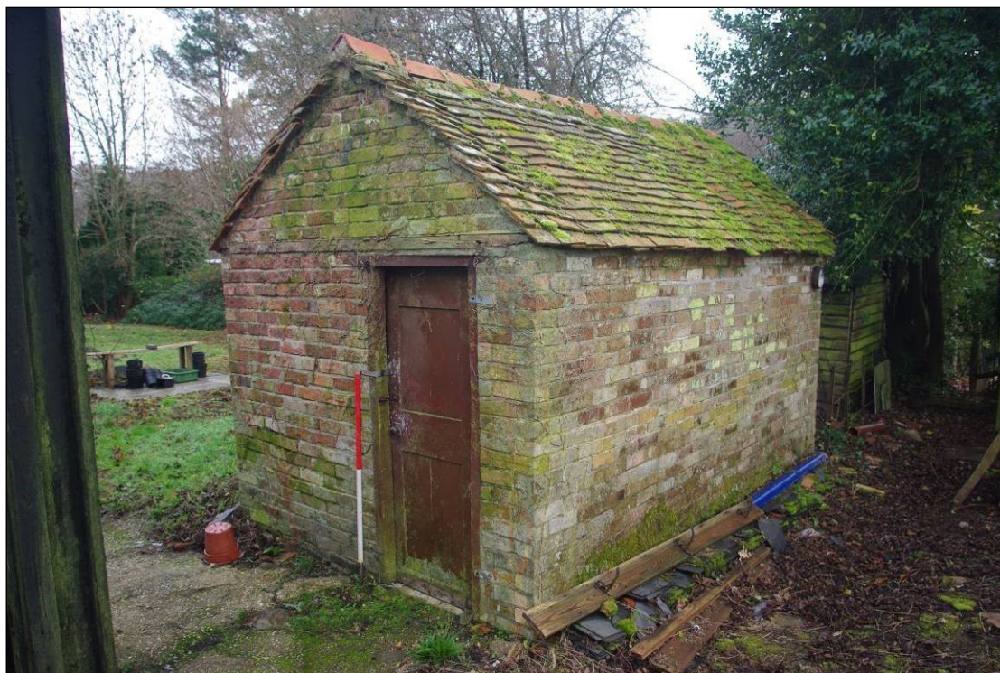
Figure 24. Room 11 external brick shed, from the northwest.
