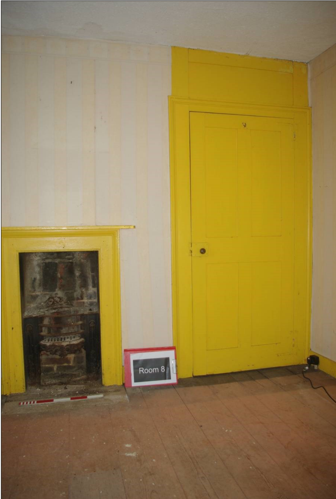
Figure 20. South wall of Room 8 with fireplace and built-in cupboard.
