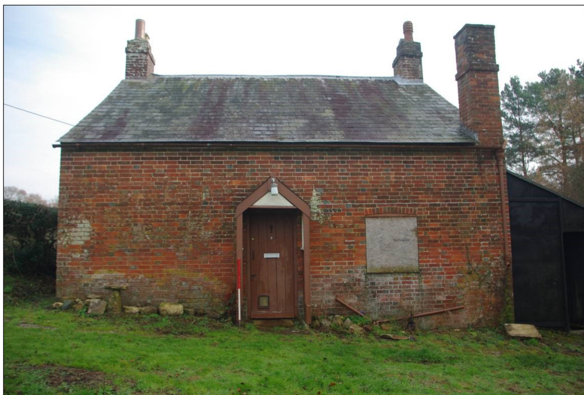
Figure 3. West elevation (rear). Right hand single stack for copper in scullery.
