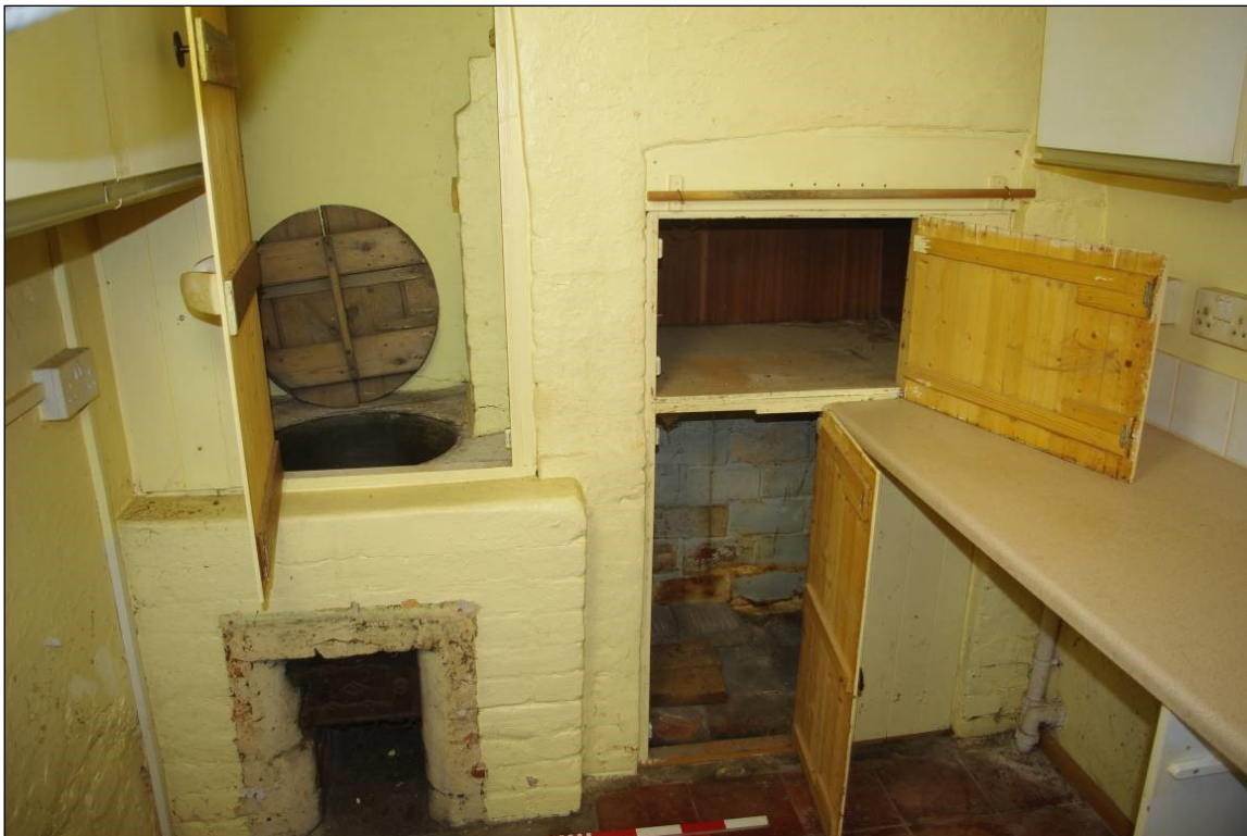
Figure 14. Copper and cupboard in south wall of Room 4.
