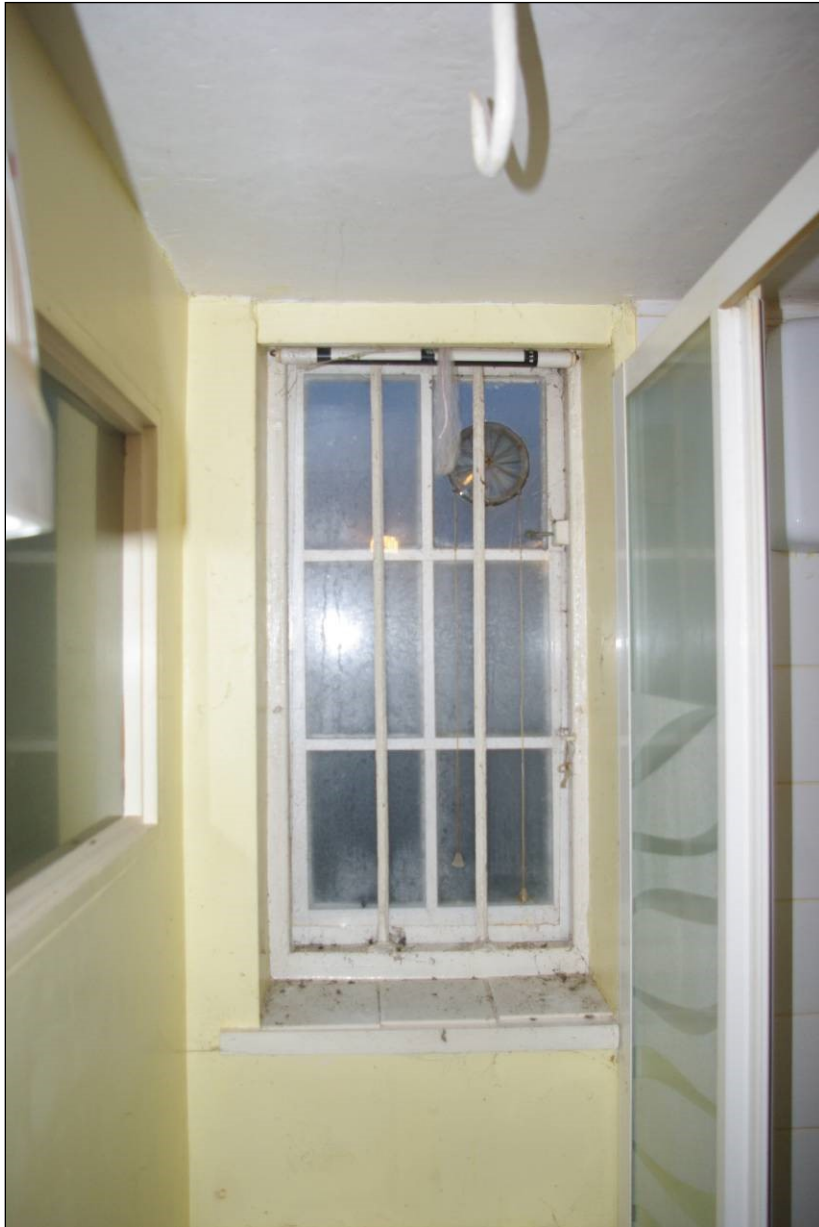
Figure 15. Barred window and carcass hanging hook in ceiling in room 5.
