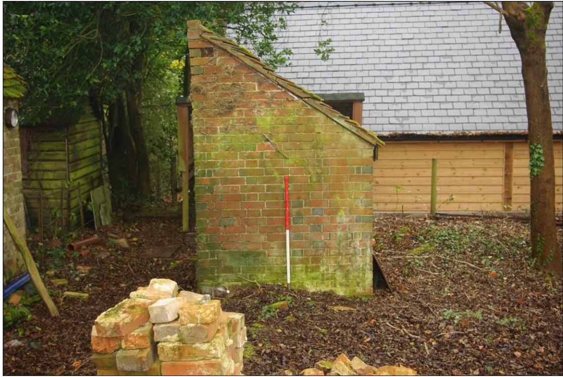
Figure 26. Brick earth-closet, Room 12, from north.
