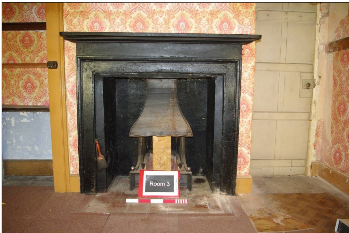
Figure 9. Fireplace in Room 3, in original opening for the range.
