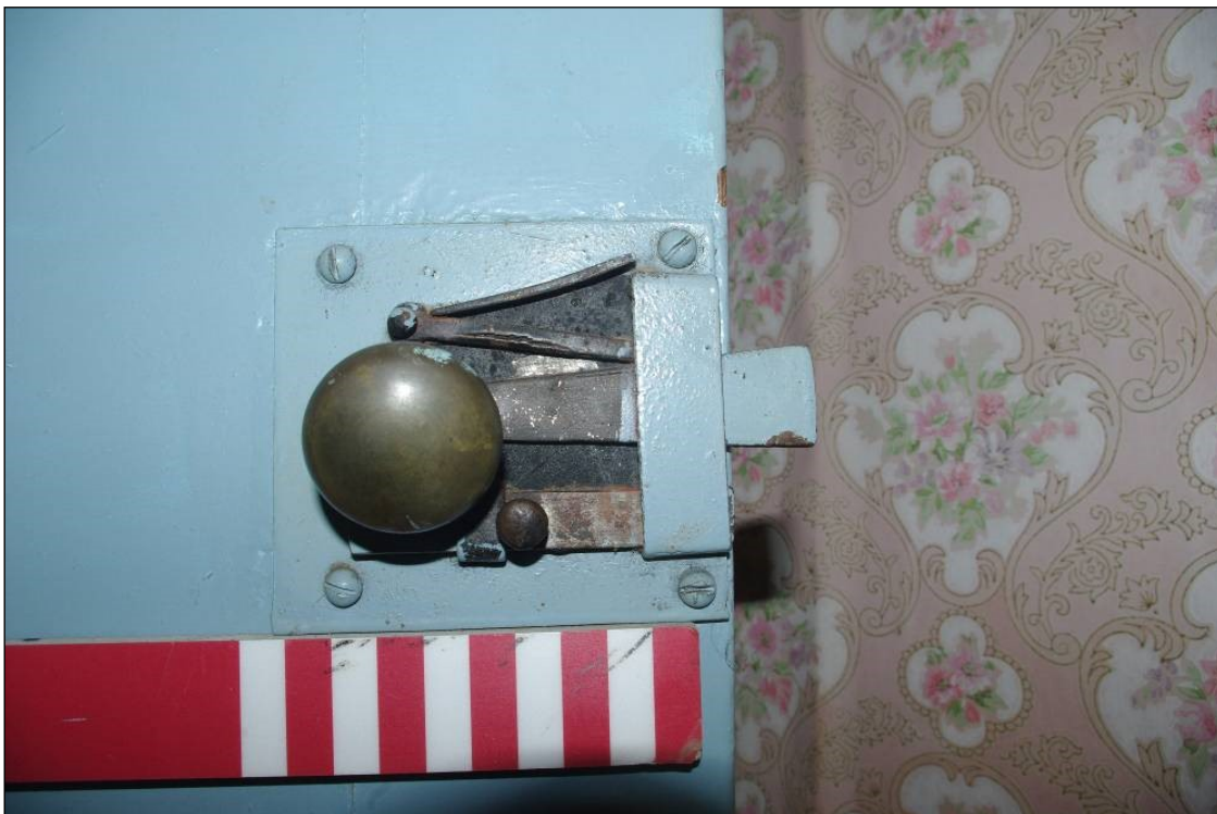
Figure 18. Door latch with privacy lock in Room 7.
