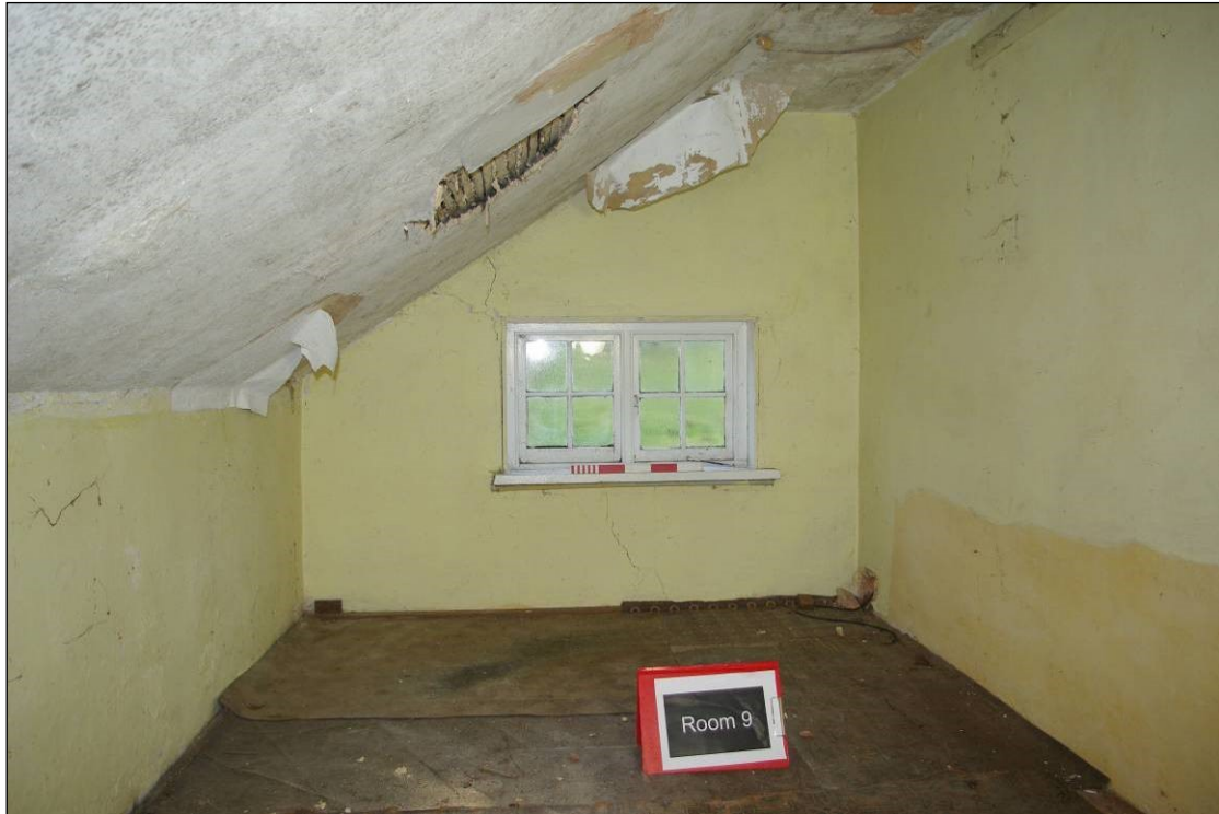
Figure 21. North wall of Room 9, beneath the cat-slide roof.
