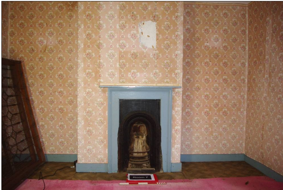
Figure 17. North wall of Room 7.
