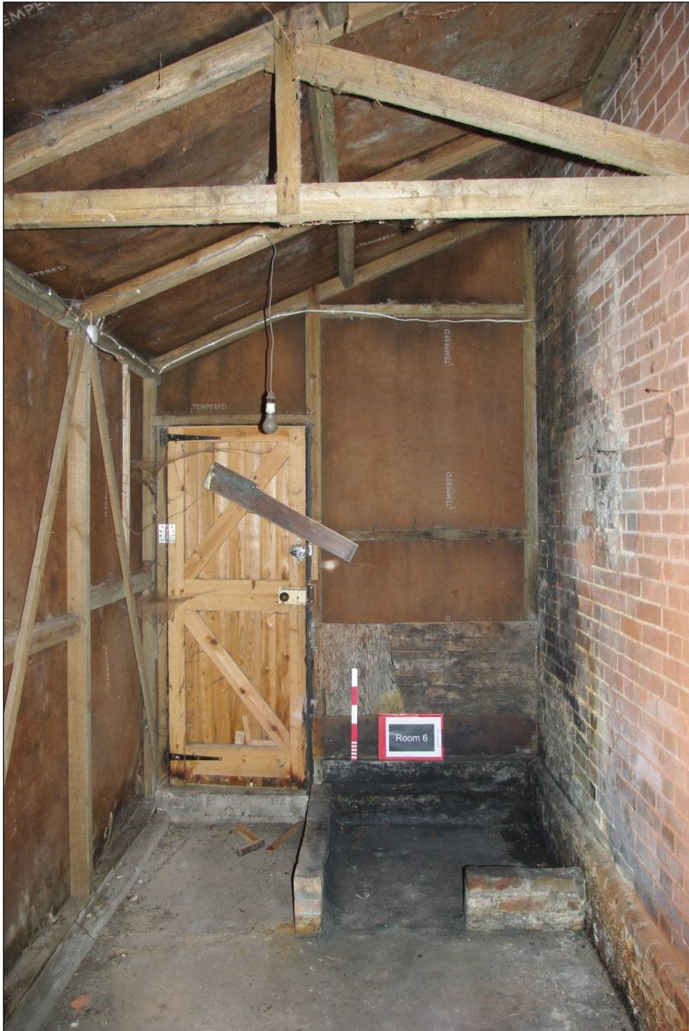
Figure 16. Room 6 looking west.
