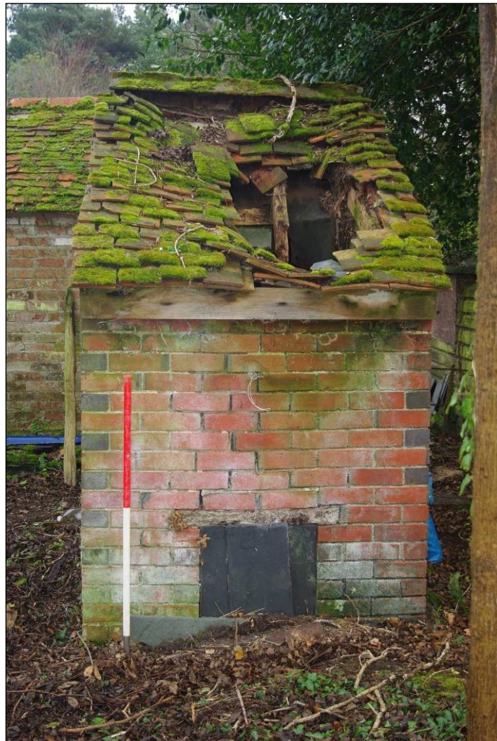
Figure 27. Brick earth-closet, Room 12 from west, showing opening for emptying bucket.
