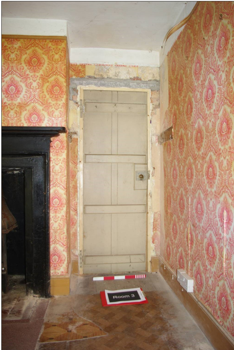
Figure 11. Door from Room 3 to Room 6, recently inserted, and originally in Room 10.
