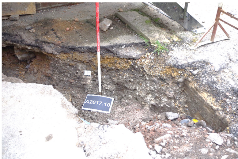
Figure 5. Drainage trench immediately behind the Vine Inn (Area 1).
