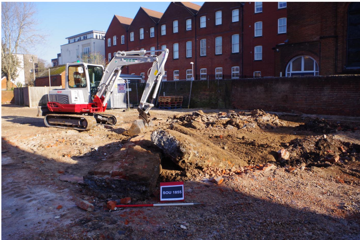
Plate 2. View of trench 1 looking northeast, showing context 4.
