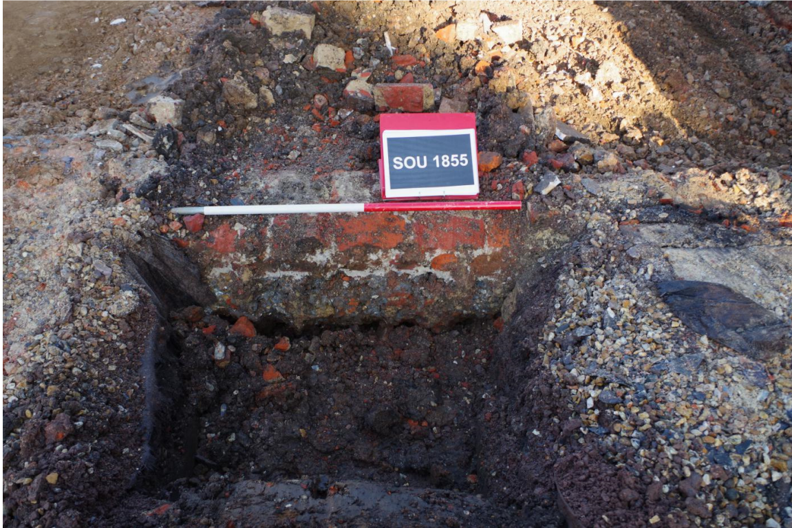
Plate 1. South-facing section of Foundation 4.
