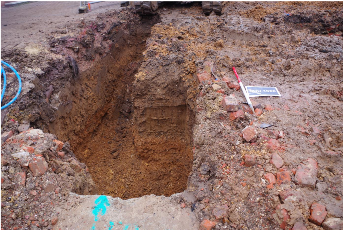
Plate 5. View of Trench 7, looking north, showing the River Terrace gravel in the base of the trench.
