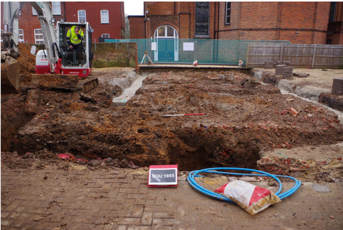
Plate 6. Overview of site showing foundation trenches near completion.
