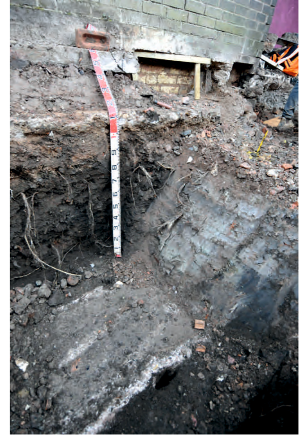
Note imported blue-grey clay infill over concrete
