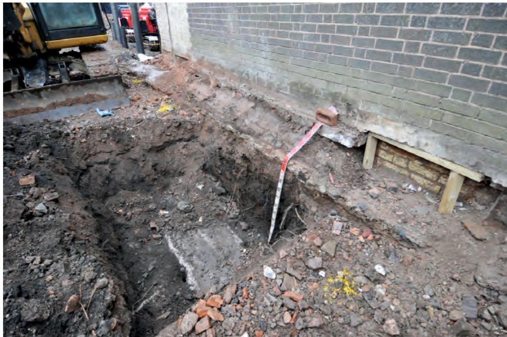
Area of deepest excavation
