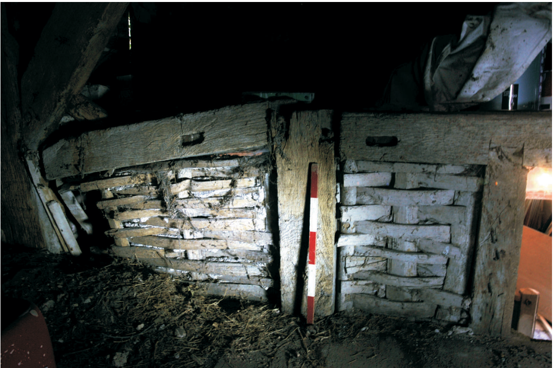
Detail of woven infill panels in internal partition wall at hayloft level
