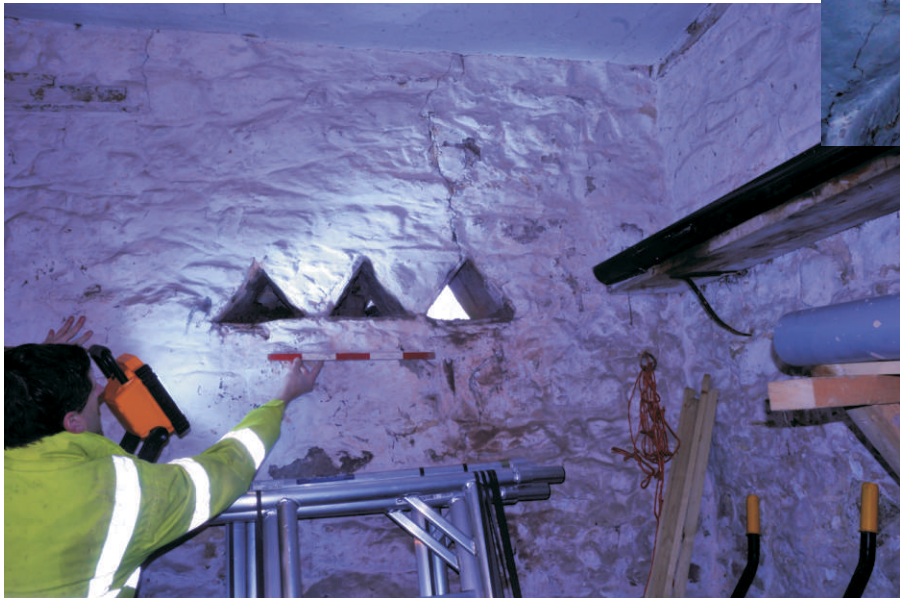
Detail of triangular vents
