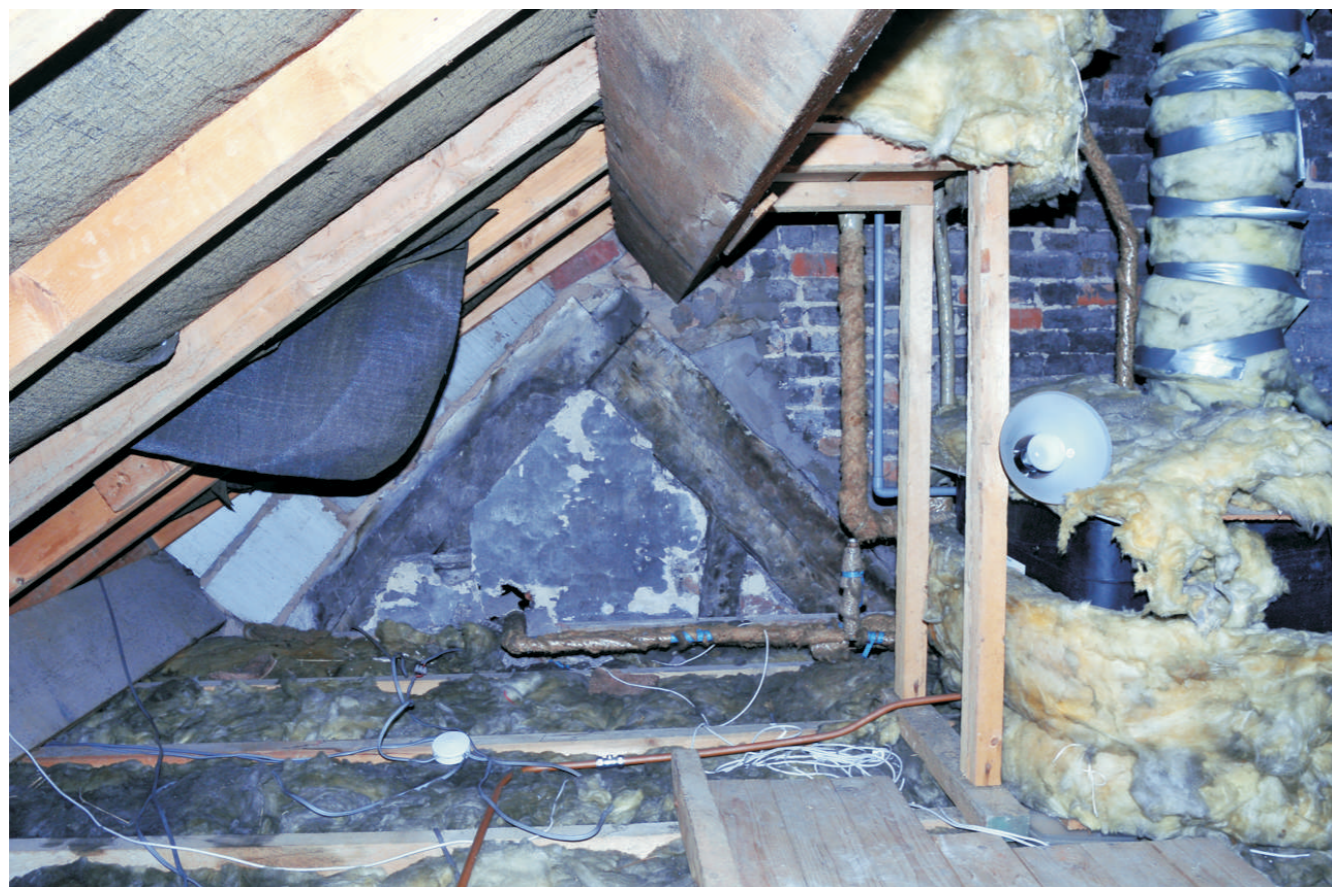
Truss 4 within the roofspace of Building 2
