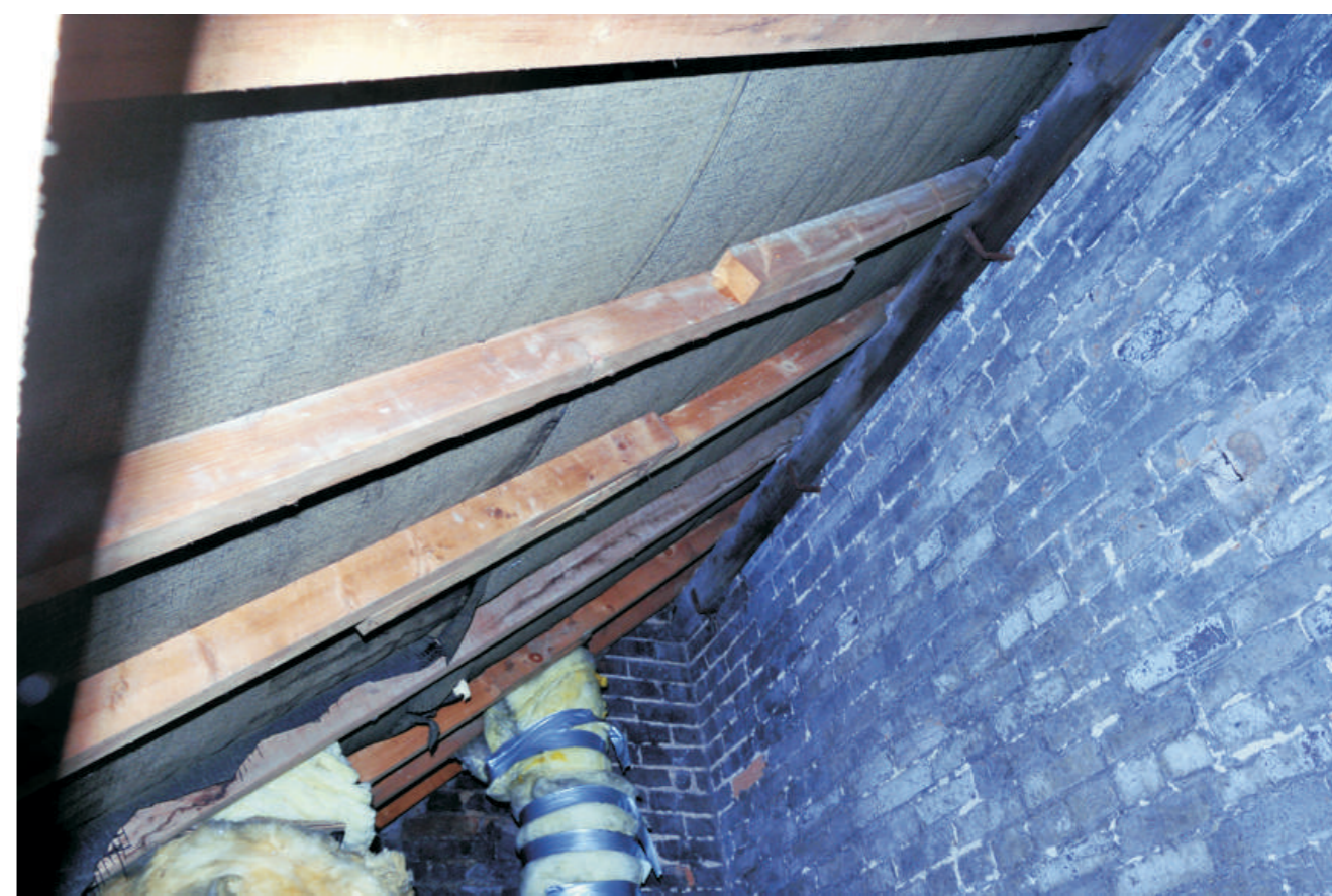
Lodging of modern Building 2 roof on earlier timber spiked to rear wall of Building 3
