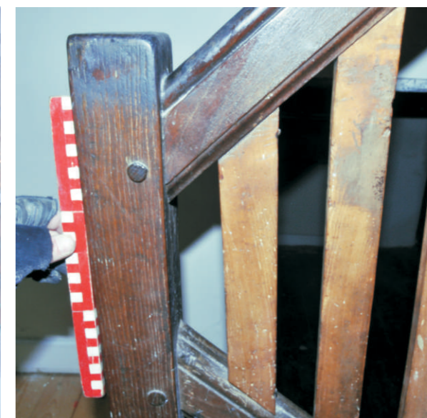
Detail of stair rail (balusters are recent insertion)
