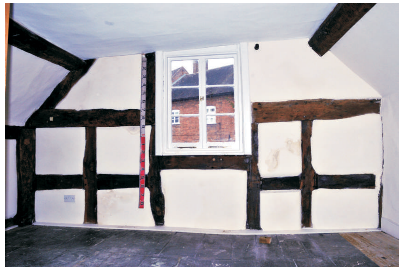
Interior of Truss 3
