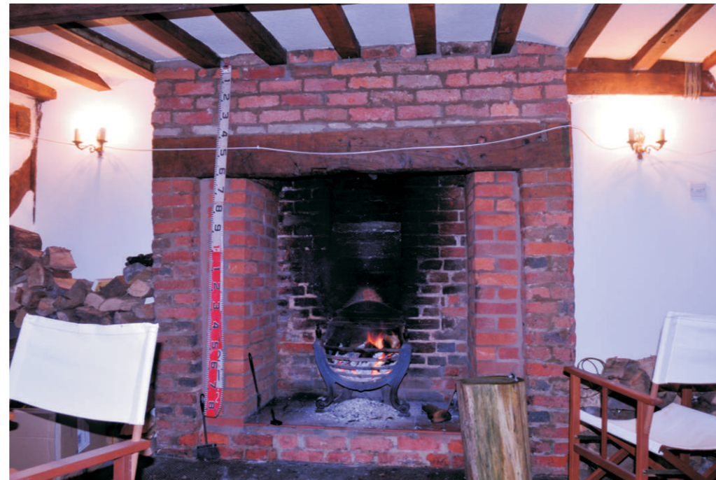
Modified inserted late 18th C chimney and fireplace - note reduced floor level around hearth
