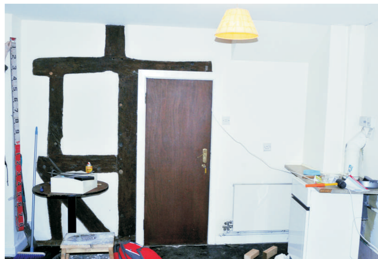
Framing of Building 1 visible from kitchen of Building 2
