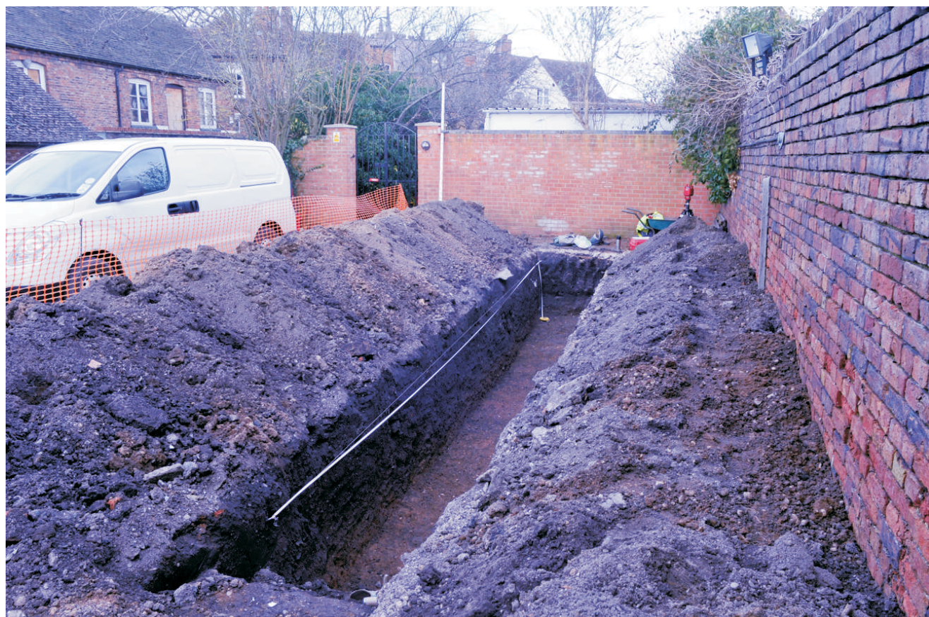
View of trench facing north
