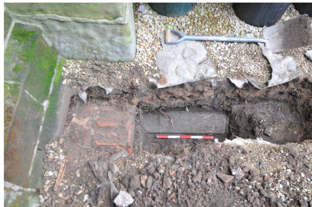
Figure 4: Exterior trenching - note chamfer course of ashlar extending 3m south of tower and representing earlier west wall of aisle
