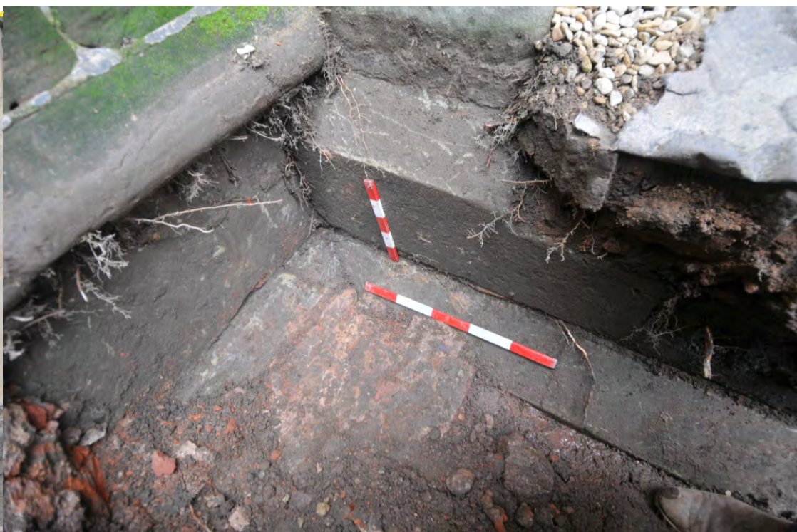
Detail of lower chamfer continuing around tower and along stub of wall
