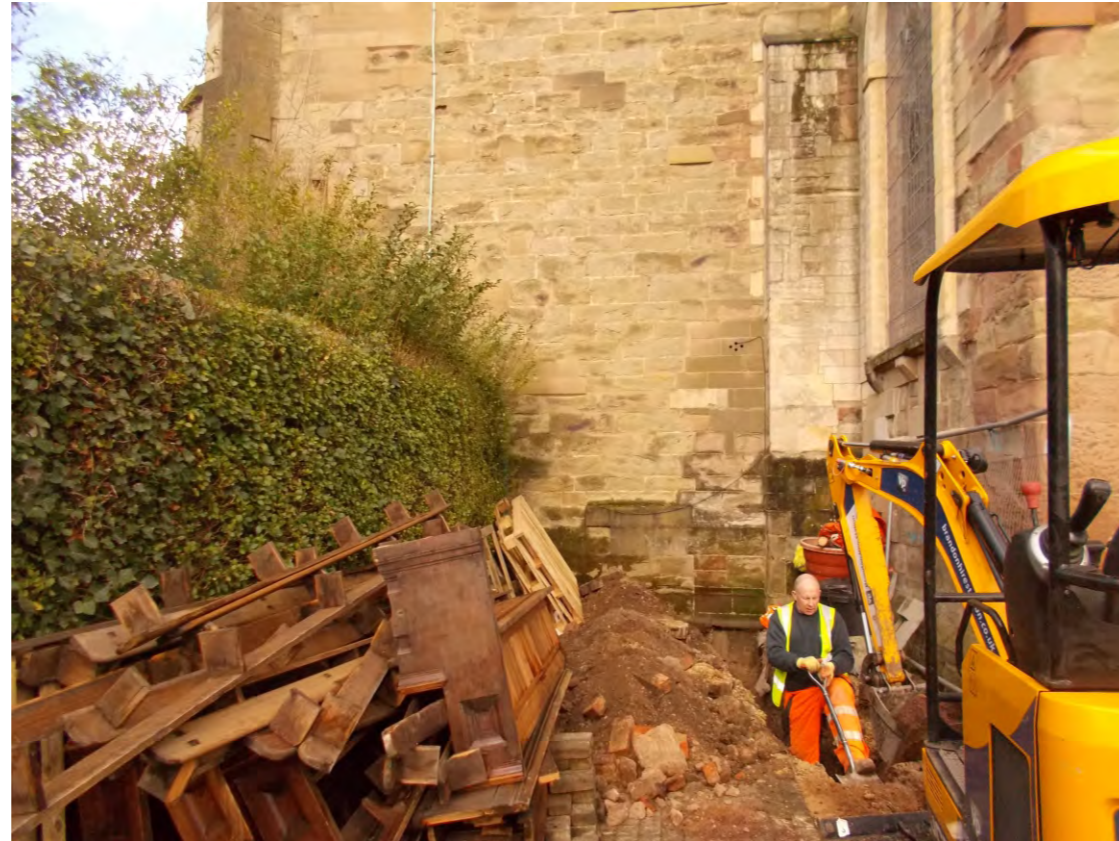
View facing north
