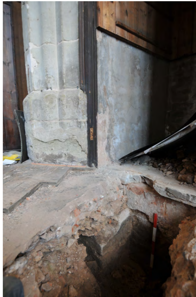
Detail of ashlar return; possible former chancel arch
