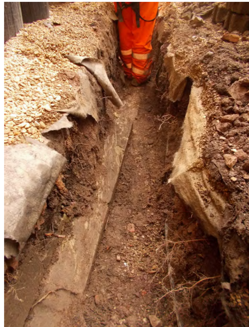
View south along stone foundation
